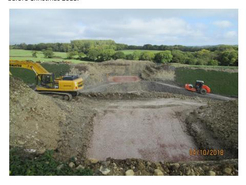
A significant section of work has also been commenced at the southern end, Hawking Centre to Waycock roundabout. Here the asymmetric widening has recently started with all trees cleared and the earthworks operation is now ongoing. To complete this section of work there will be the need for various road closures which will be communicated in advance once approved.
