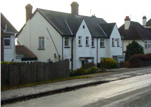
Houses stand below the road level to the south of Porth-y-Castell.
