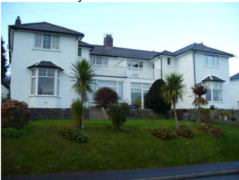
Houses on the north side of Porth-y-Castell with balconies to exploit the views.
