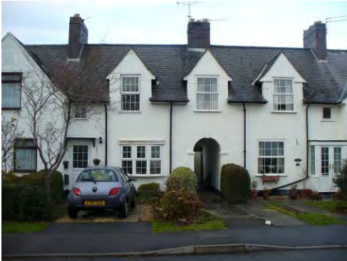
Short terrace of cottages on Westward Rise.
