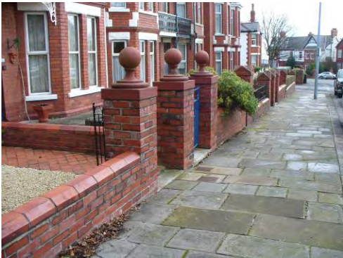
Flagged paving and brick boundary walls on Park Road.
