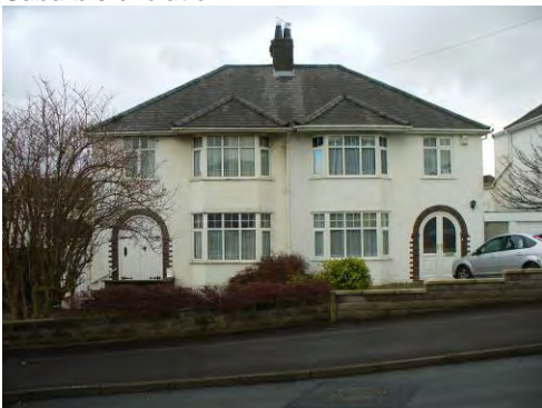
Houses built to the designs of the Great Western Railway in the 1920s
