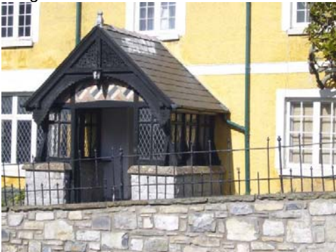
Porch and historic railings at Boverton House.
