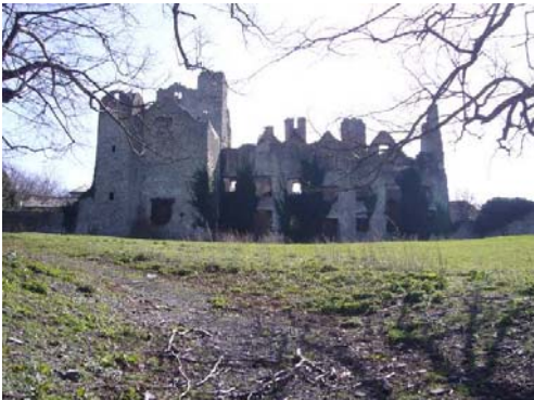
Boverton Place, a picturesque ruin above the village centre.
