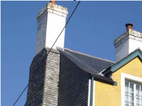
Slate hanging on the western gable of Boverton House
