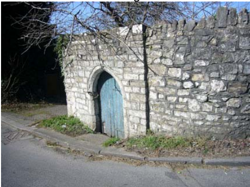
Walls Surrounding Garden West of Boverton House
