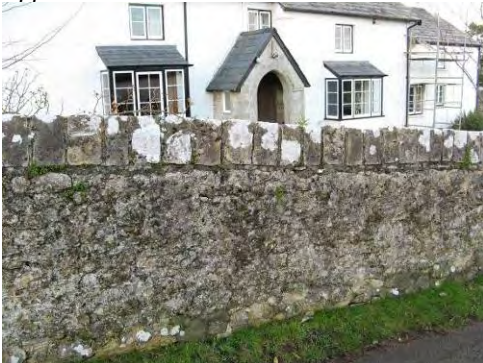
Stone walls outside Y Hen Fferm Dy.
