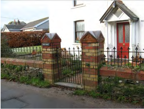
Original railings and gate set in brick piers at High Croft.
