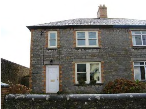
Modern, but well detailed windows on Windways.
