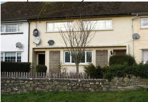
Here a large number of satellite dishes dilute the character of the area.
