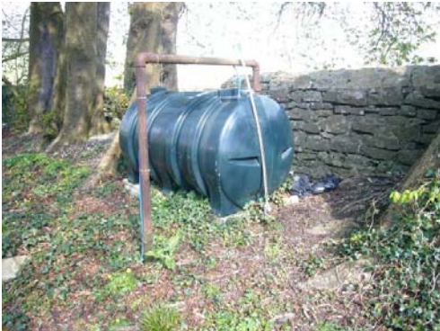
This oil tank might be concealed by a screen.
