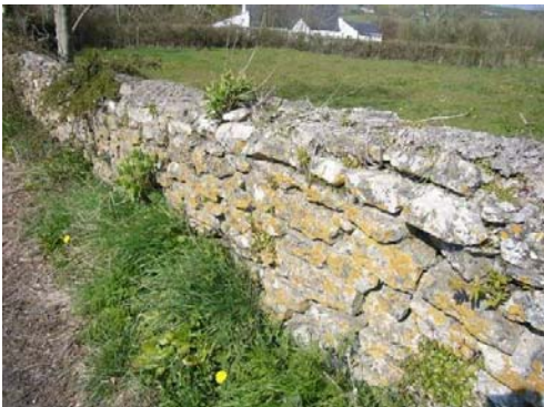
The stone wall between Church Farm and the Church.
