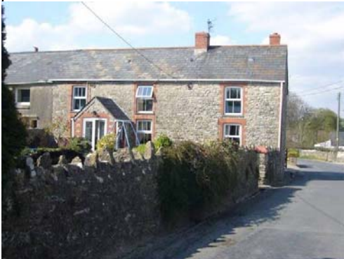
The use of red brick suggests that this building was constructed in the 19 th century.
