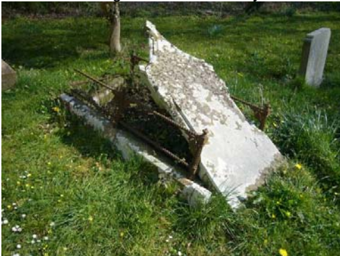
Some gravestones are in need of attention.
