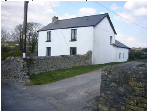
Stone walls are a distinctive feature of the conservation area.
