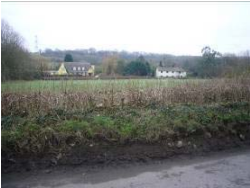
Part of the enclosure of the area's central field. Note the damage to the grass bank done by vehicles
