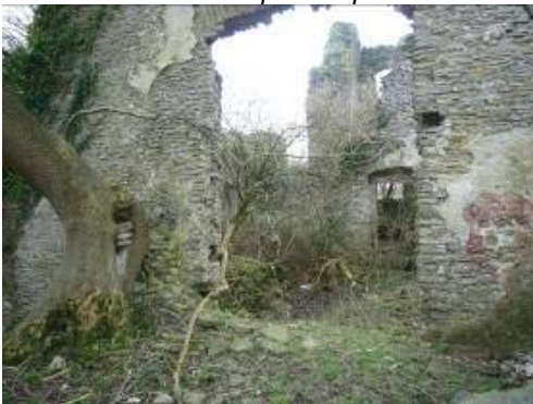
The ruins of Llantrithyd Place are in need of stabilisation.
