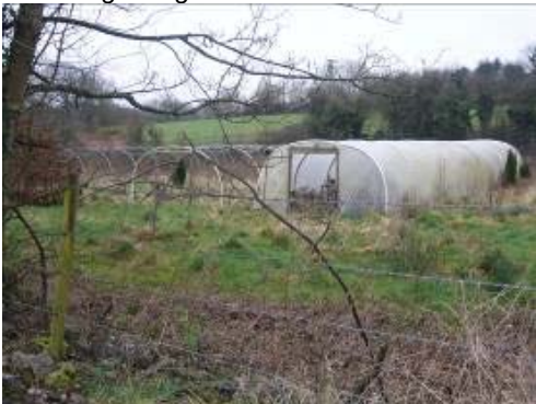
Disused polythene tunnels are unsightly.
