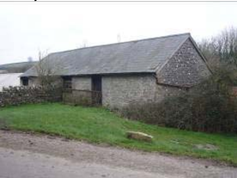
Agricultural building built with local lias stone and slate roof.
