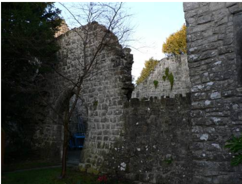
The ruinous Chapel at the western end of the Parish Church.
