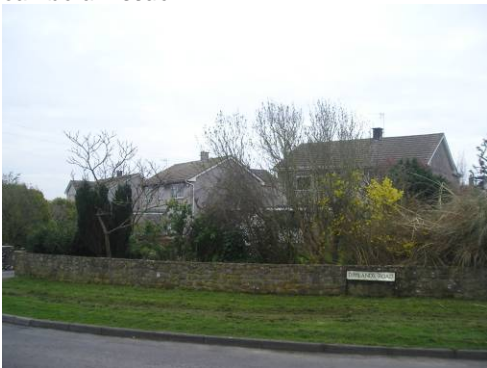
There are examples of poorly considered development in the Conservation Area.
