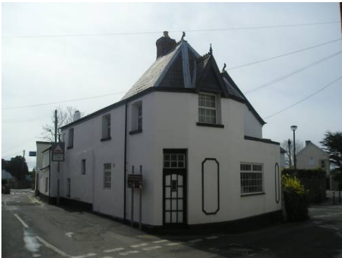
Many buildings sit directly on the road, or against narrow pavements.
