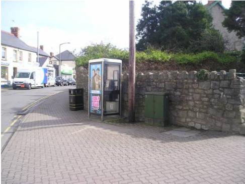
In places, the public realm is of a poor quality and there may be potential for improvements.
