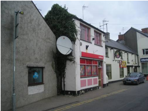
There are examples of poor quality shop fronts.
