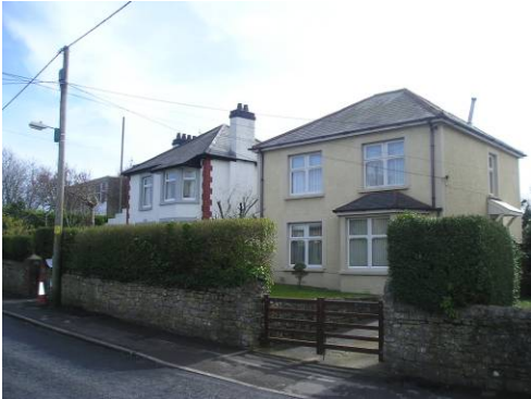
Modern development and inappropriate alterations to buildings on Station Road have diluted the character of the Conservation Area.
