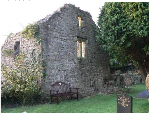
Former Chantry Priest's House.
