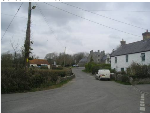
Wider roads and more dispersed buildings are evident here where the town gives way to the surrounding countryside.
