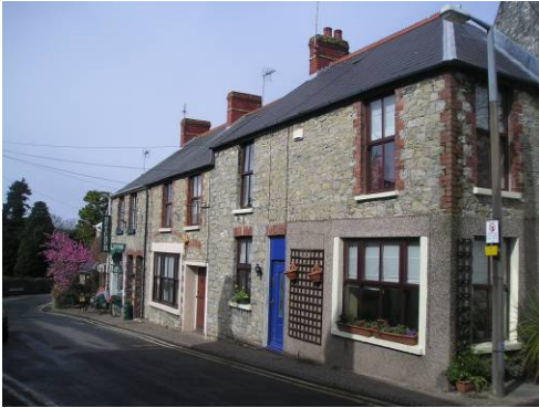
There is evidence of former commercial uses in these houses on Church Street.
