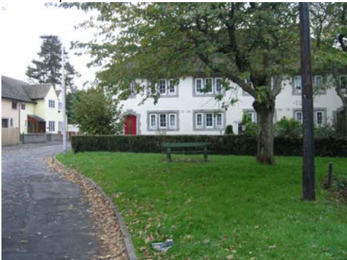
Former Rural District Council Housing at Croft John is an important element.
