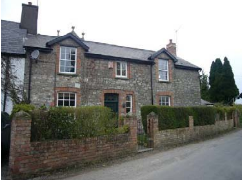
Springfield has red brick dressing around its windows and doors.
