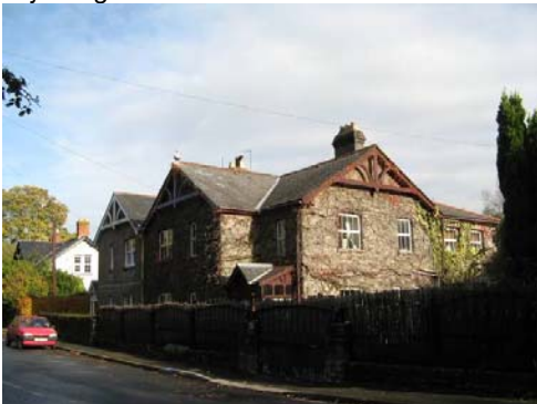
Former Estate houses in Old Port Road (nos. 13 and 15).
