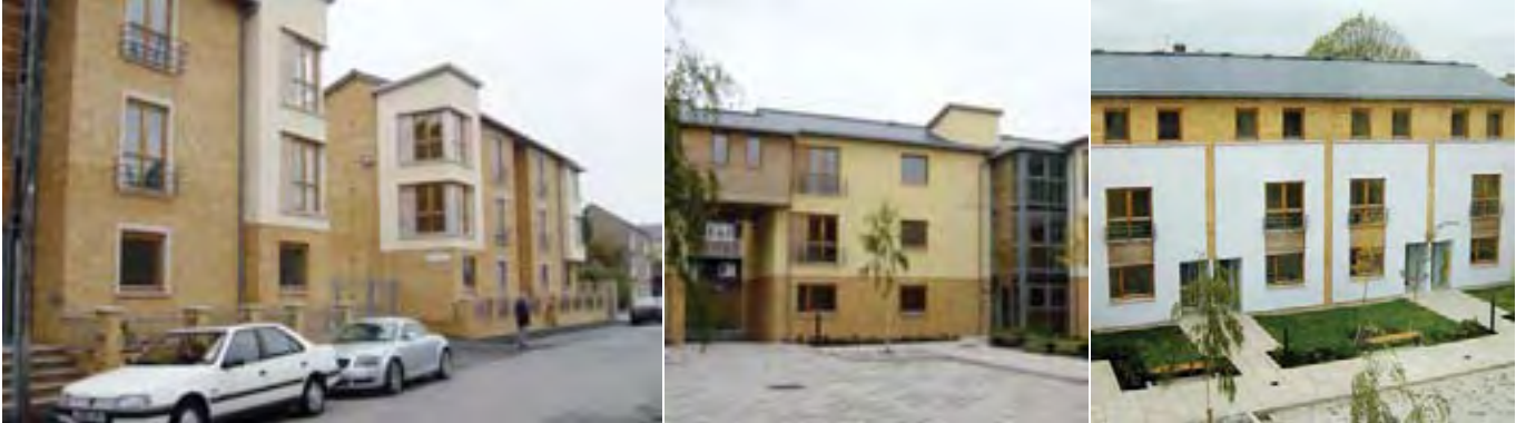
INSIDE AND OUT: STEFFANI COURT: PCKO/PENTAN
