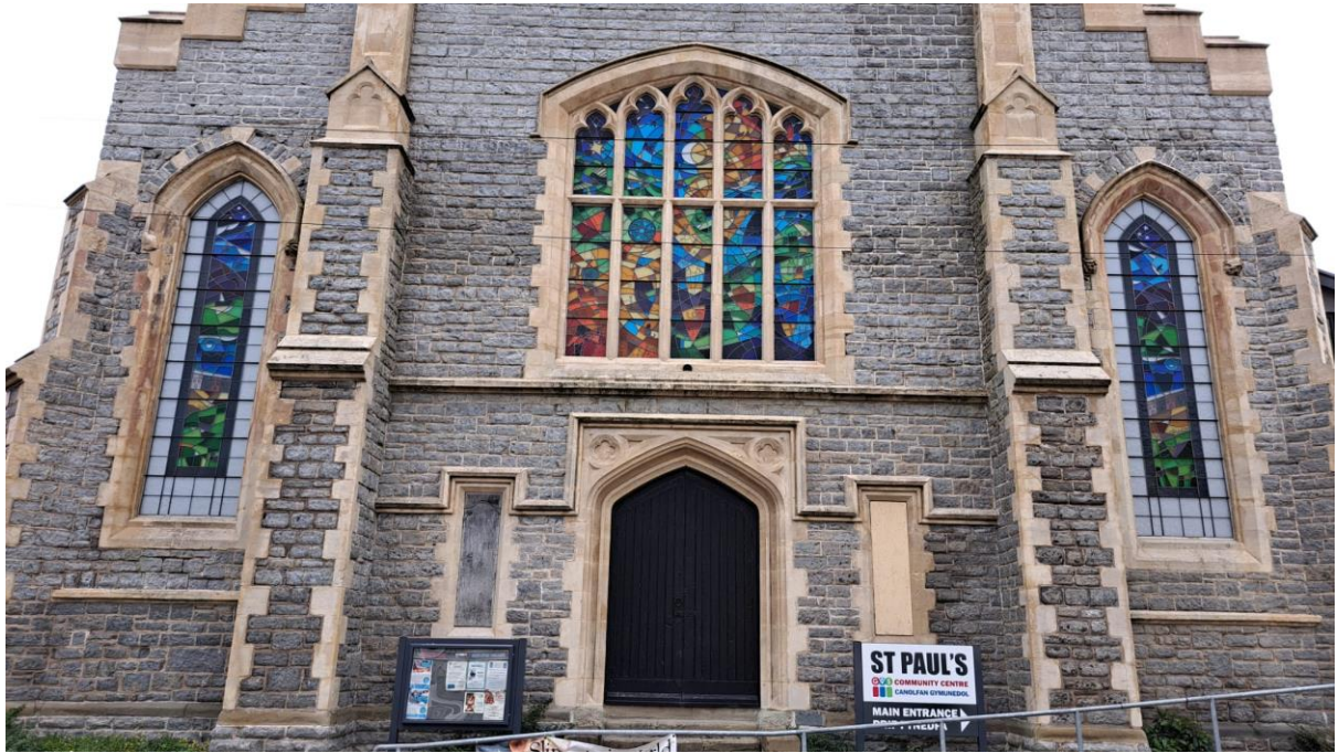
Completed main central window and side windows
