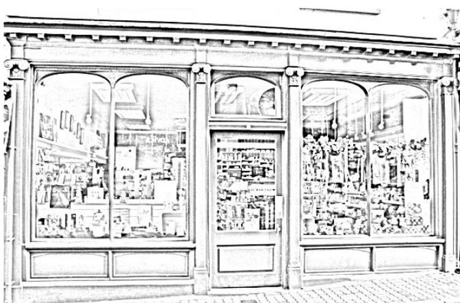
*A row of several shops in Cowbridge, all have stall risers for structure, balance, and protection from damage.*
