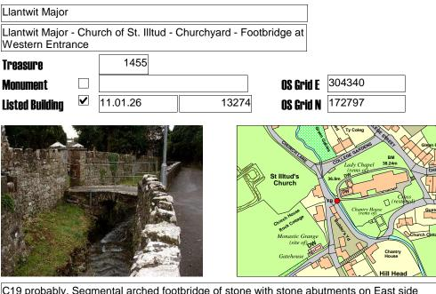
C19 probably. Segmental arched footbridge of stone with stone abutments on East side and flat modern concrete deck. C19 iron rail balustrade, terminating in square uprights with pyramidal finials.
