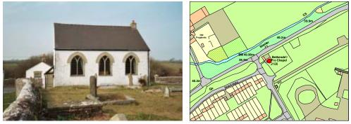
1807 noted non-conformist chapel, rubble, slate roof, eaves end gables. One stone end stack. Plain square head door in South West elevation, slated pentice hood on wooden supports. South East long elevation has three pointed arch windows with forked mullions, two light with lead panes. One of the greatest Welsh hymn writers of the C18, Thomas Williams, was minister at this chapel.
