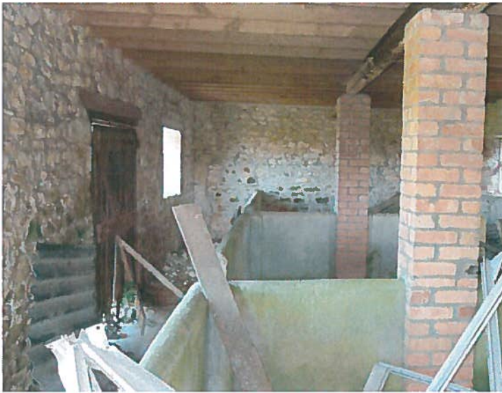
15. An interior view showing the pens and the inserted structure
