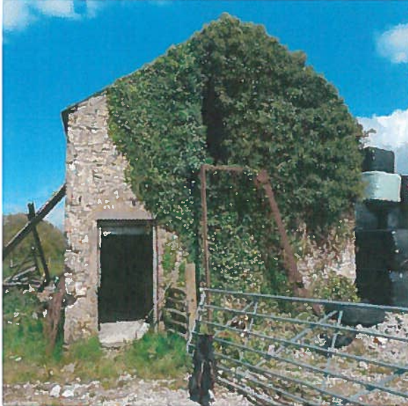
11. The South East gable.
