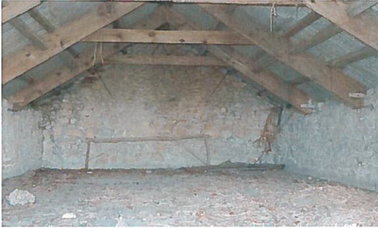
16. View of the upper storey within the roof
