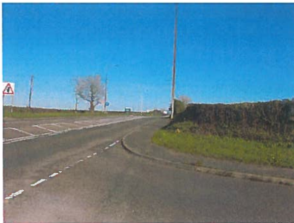
Crack Hill junction
