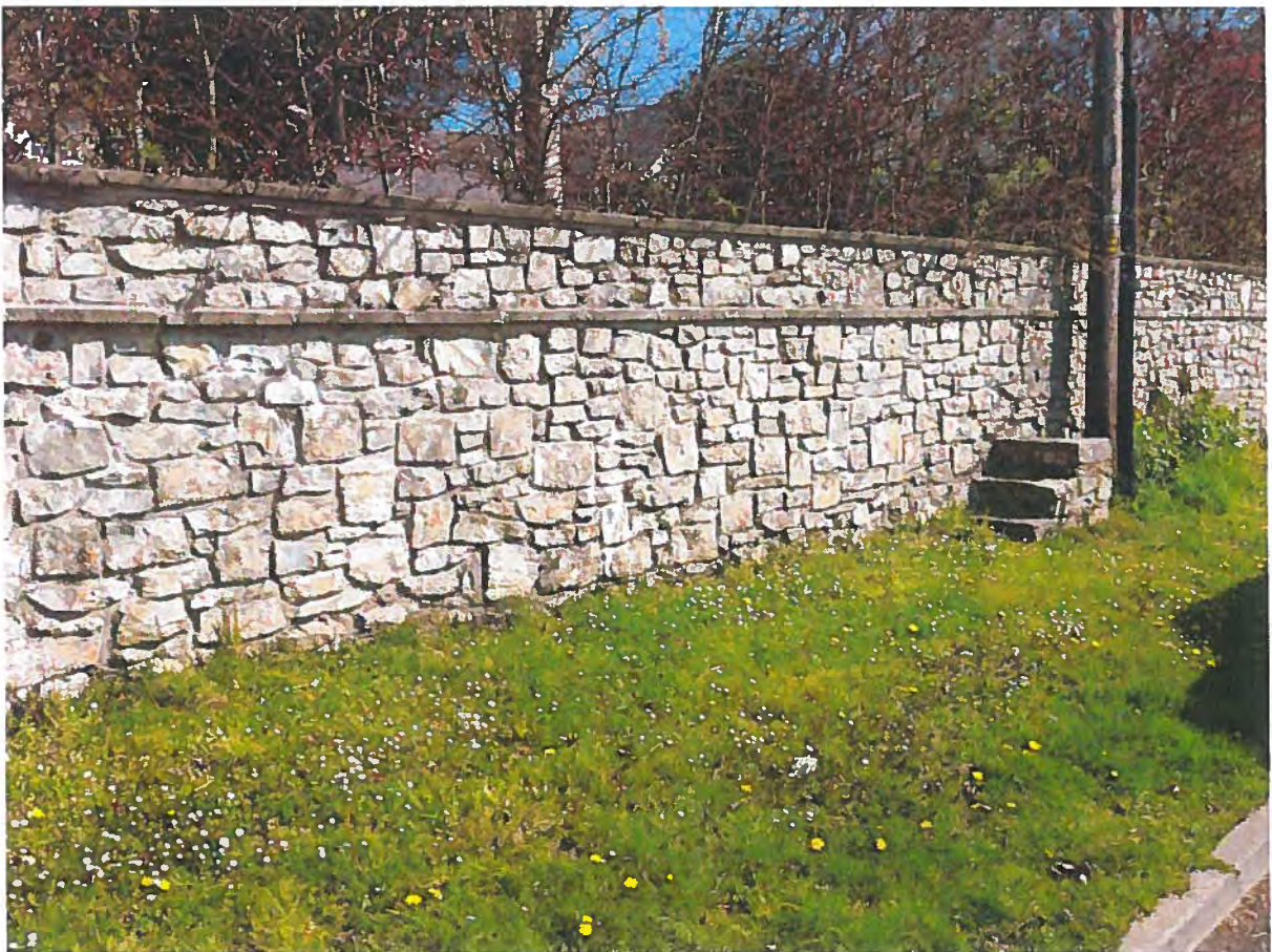
Restored stone boundary walling
