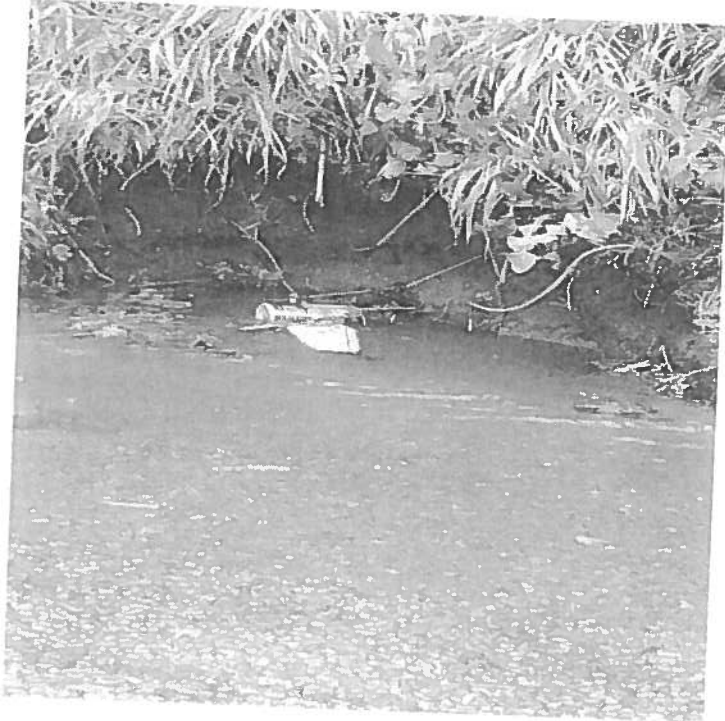
Pic 7 – storm drains further downhill from the site overflowing during a medium rain event. This flooding freezes in winter meaning the road is not passible safely. The effect of adding effluent from 39 extra residents in the area, to this already overstretched system cannot be predicted.
