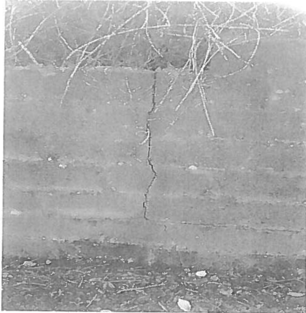
Pics 4 and 5: Cracks in the retaining wall downhill from the site on the Deg Erw access road. Newydd's plans fail to show how this problem will be solved safely.
