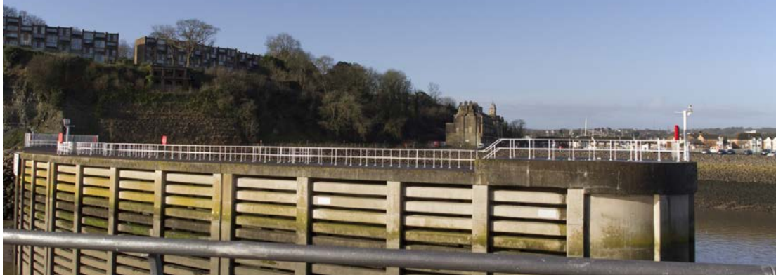
Photo montage existing
