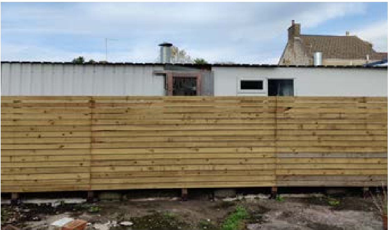
The building, which has been constructed on the boundary has now been enclosed by a fence placed immediately in front of it, as shown in the second and third photographs.
