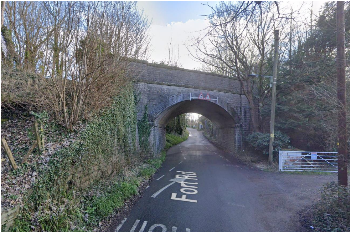
Figure 12: Viewpoint (south facing) of ATR from Fort Road
