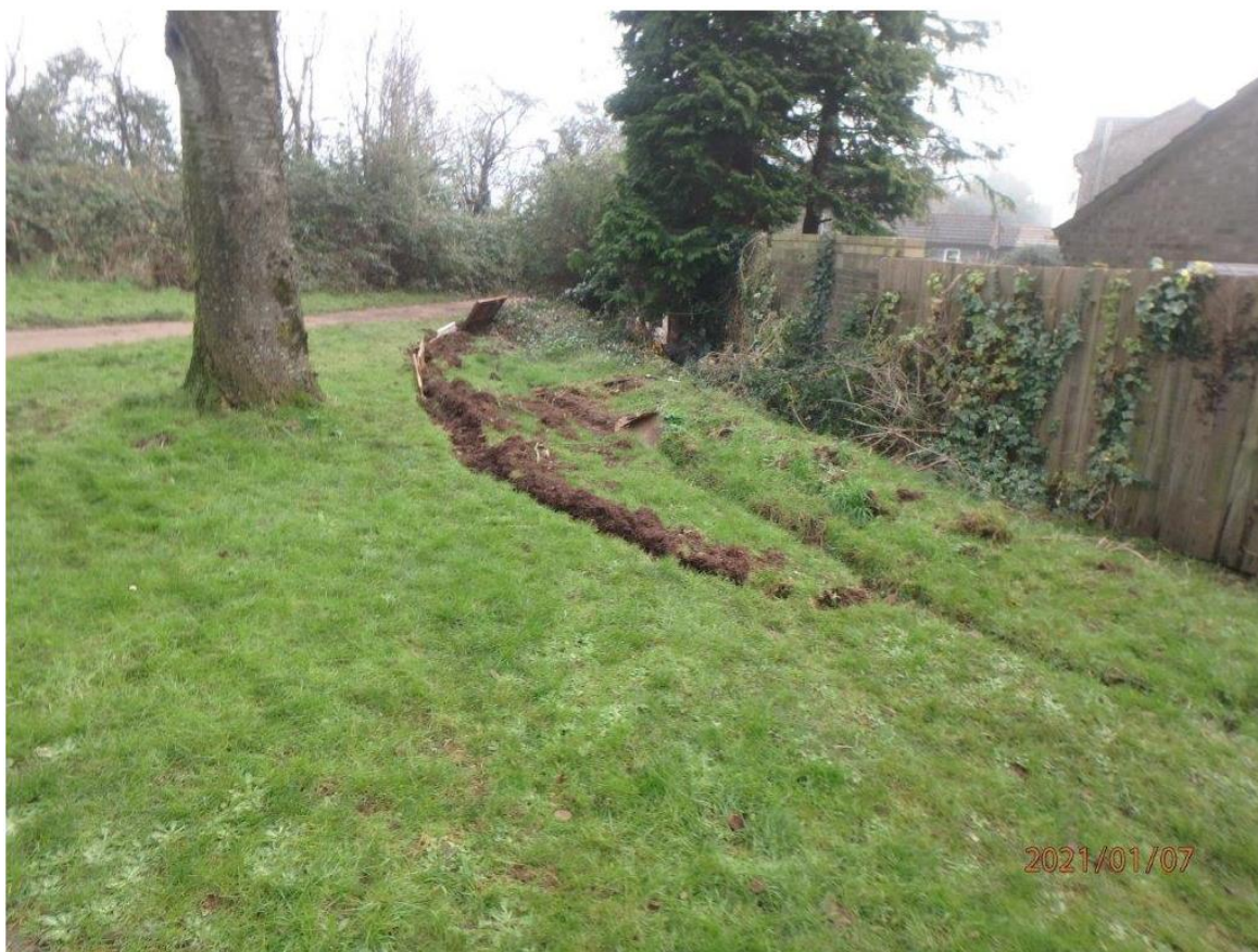
Figure 4-6 Informal defences to the rear of Conybeare Road (picture provided by VoGC)
