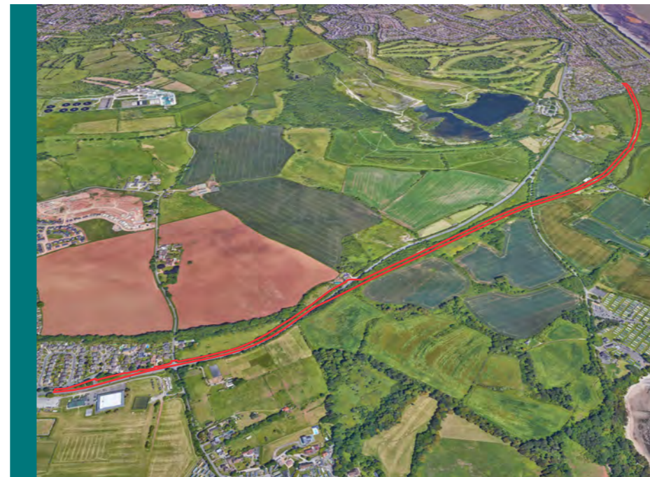
Figure 1. Location of Sully to Cosmeston ATR Site
