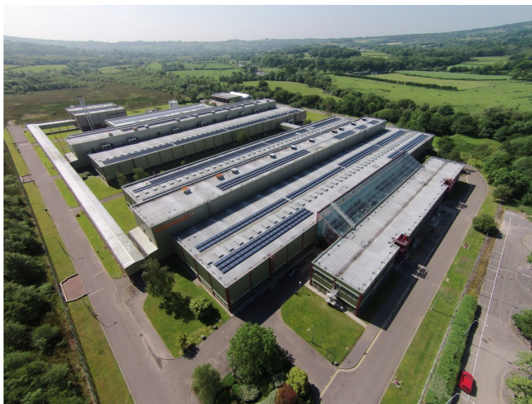
Figure 65: An example of Solar Panels used on Industrial Buildings at the Renishaw Site
