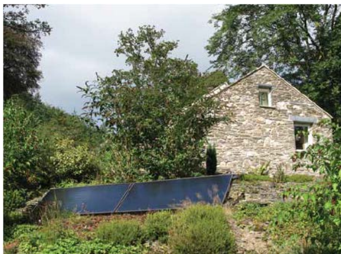
Figure 24: Free Standing Solar Panels Sited Away From an Historic Building (Source: Cadw)
