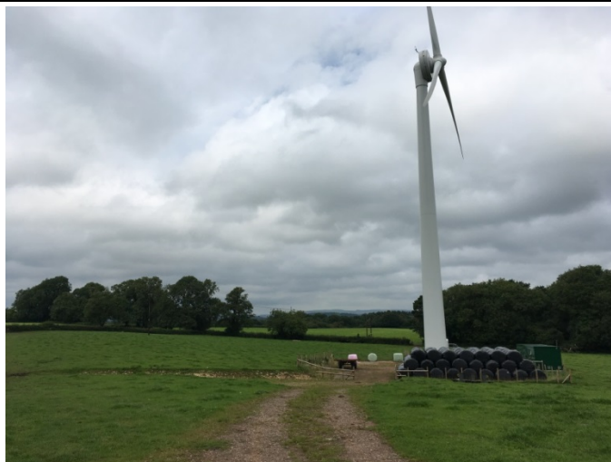
Figure 54: Example of a Medium Sized Turbine in the Vale of Glamorgan
