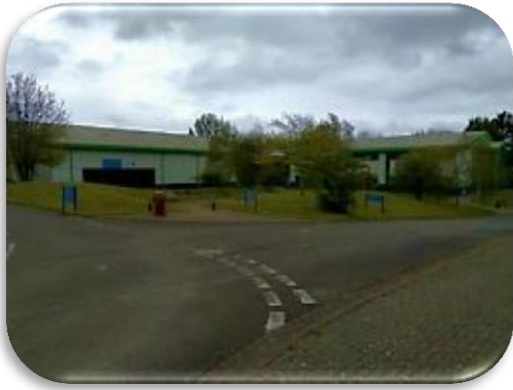
Photograph 3: View of Front of Cardiff & Vale College
