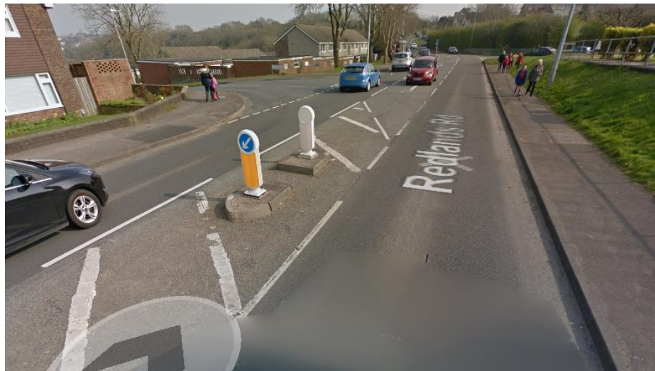
Crossing refuge provided close to junction of Foxglove Rise, though very narrow and no drop-kerbs/tactile paving.
