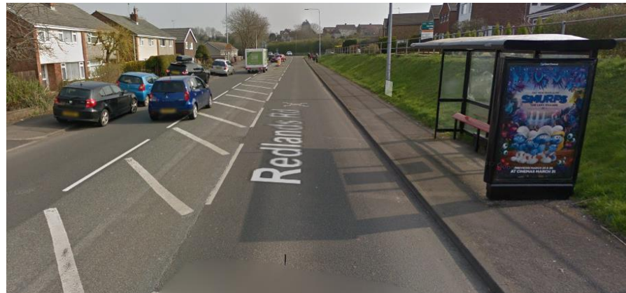
Crossing refuge provided close to junction of Foxglove Rise, though very narrow and no drop-kerbs/tactile paving.
