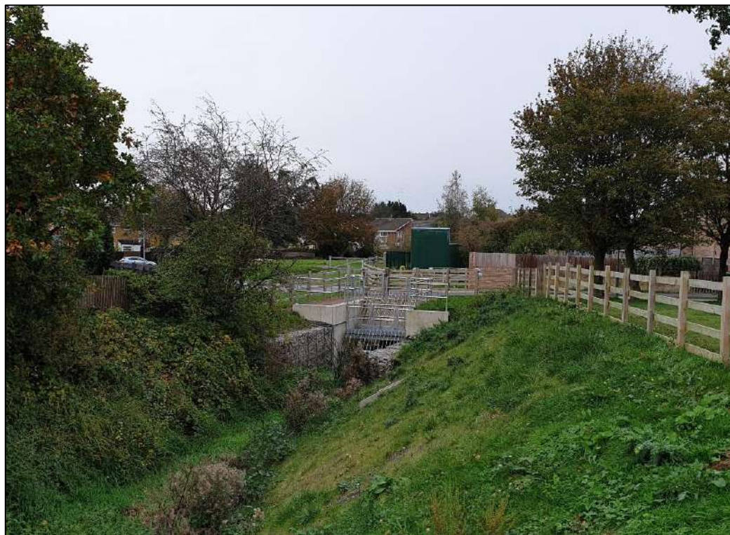
Figure 2-6: Typical Culvert Structure of the Coldbrook Flood Alleviation Scheme
