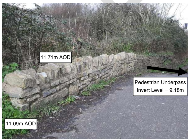
Figure 2-8: Floodwall upstream of the A4231 pedestrian underpass
