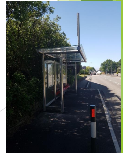
New bus stop & shelter - Ystradowen - 2019/20
