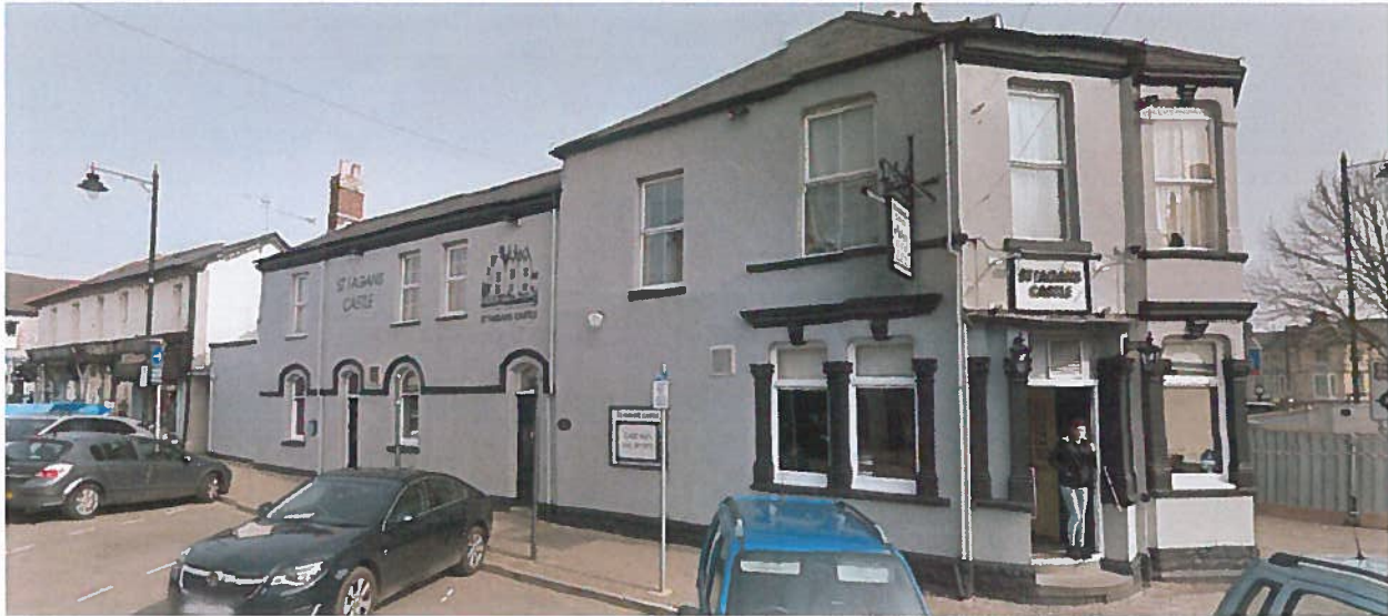
Front door to right of photo also access / egress to side door onto Glebe Street
