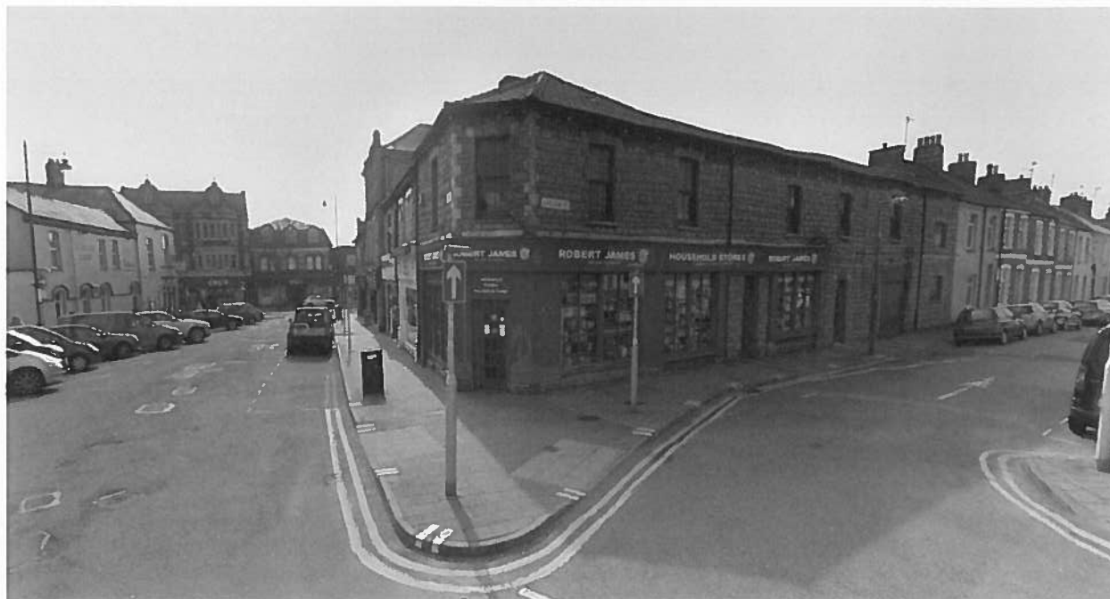
St Fagans Castle to bottom left hand corner of the photo, residential accommodation to right of photo on Ludlow Street
