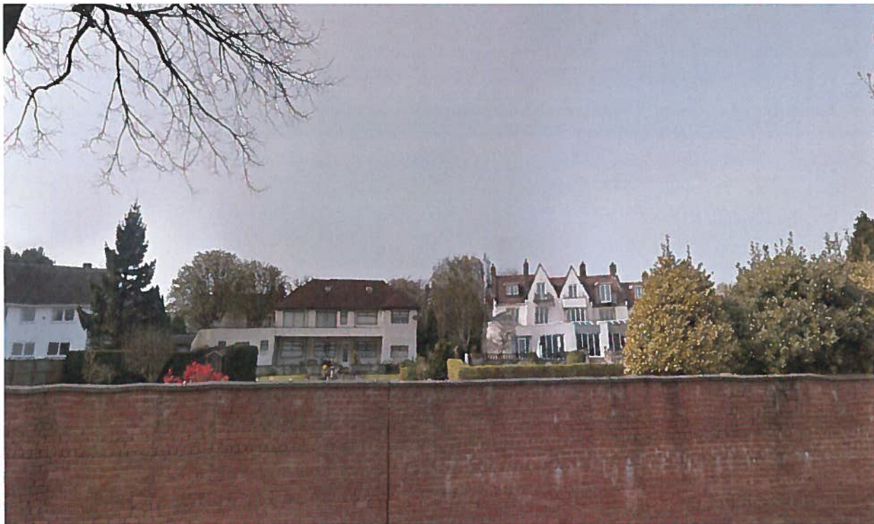
front of Holm House to right hand side of photo, bar area to be in the garden area
