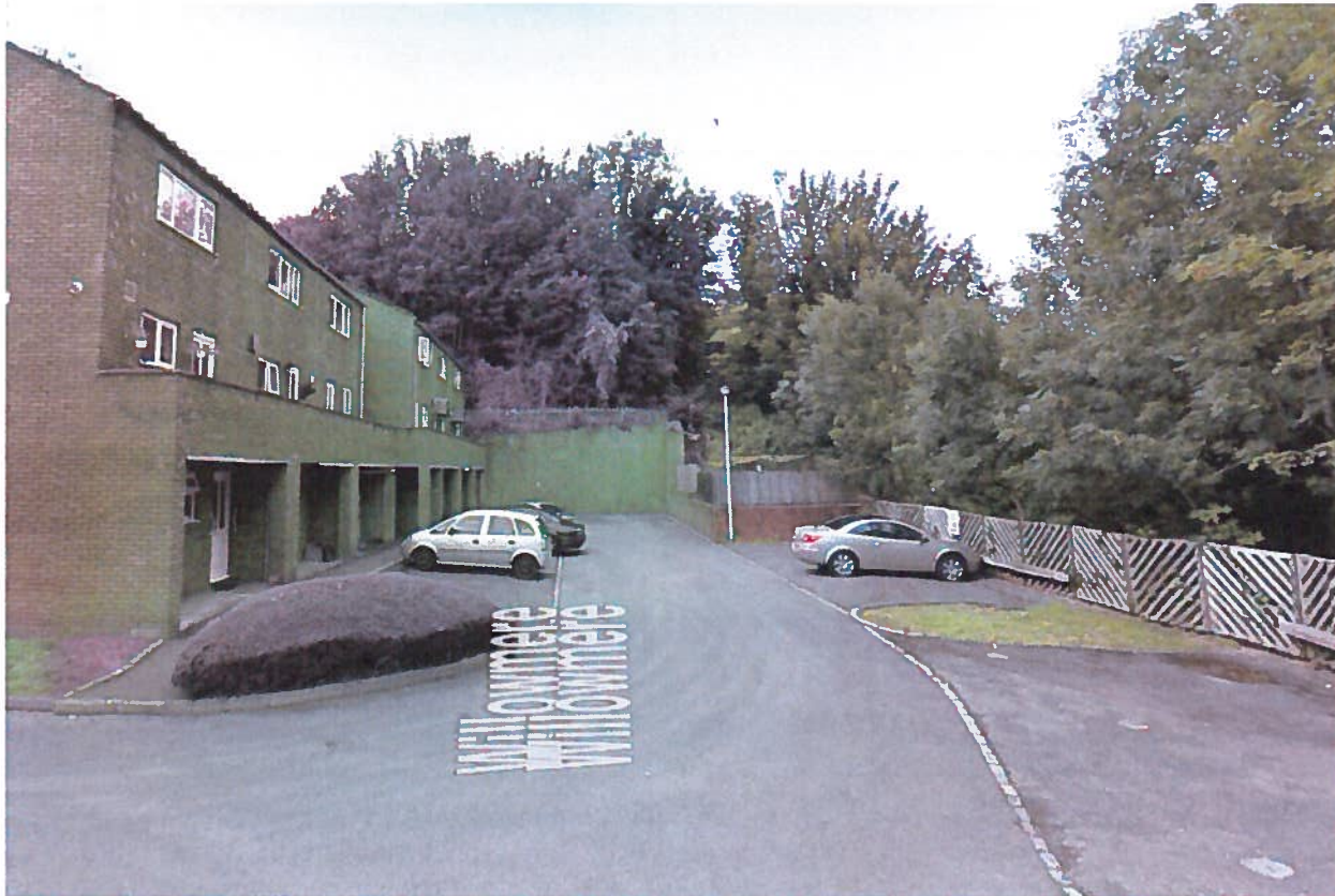
Willowmere flats overlooking Penarth Rd and the Arena.
