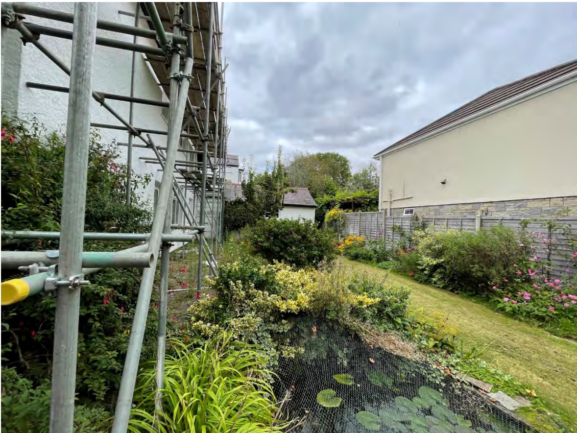
View from garden facing towards existing outbuilding
