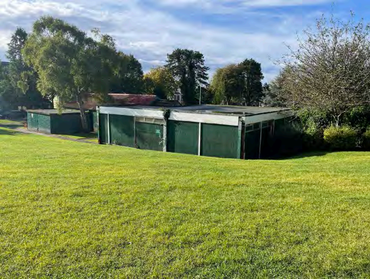
The rear of the existing building
