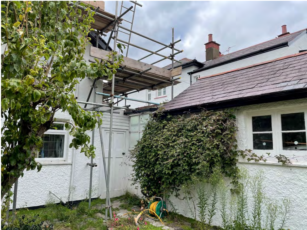
View from garden facing existing car port and outbuilding
