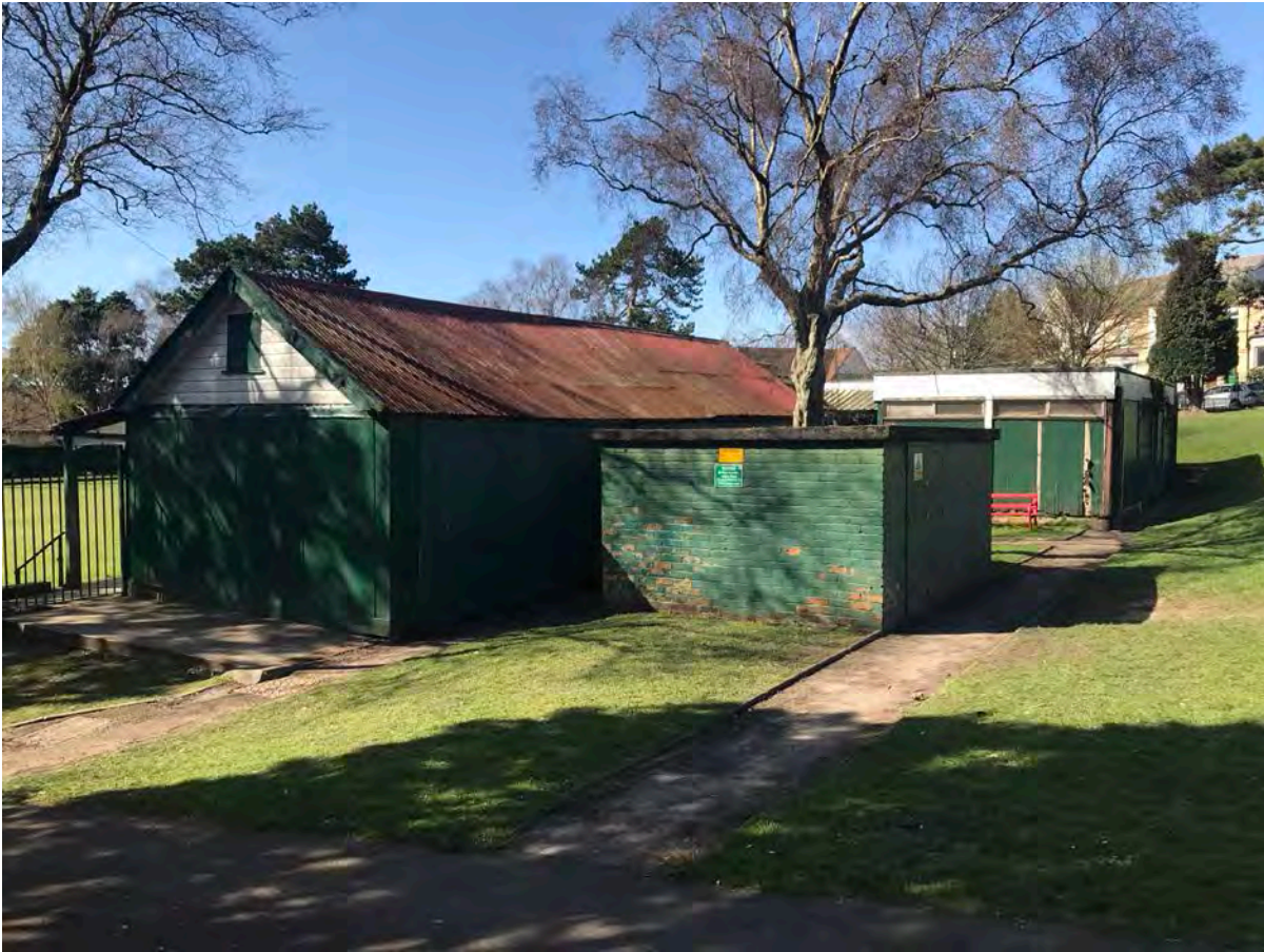
The side of the existing building
