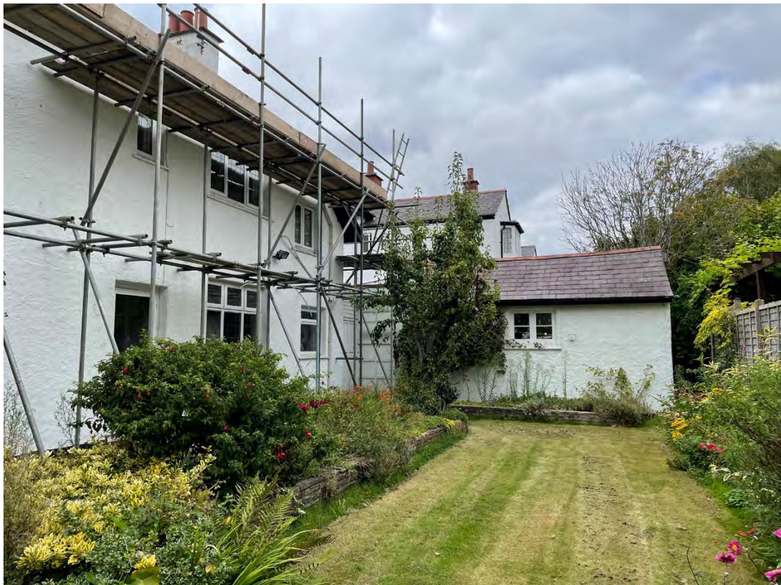
View from garden facing existing outbuilding
