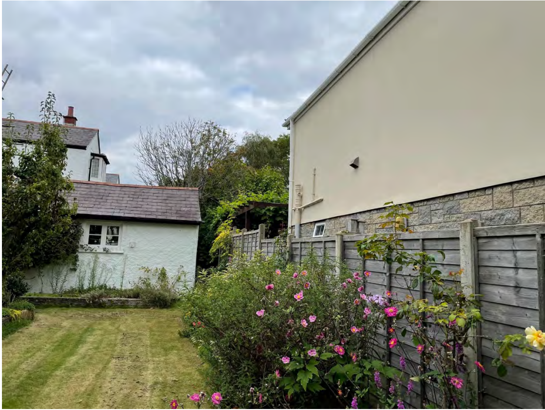
View from garden facing outbuilding and boundary with No.11a.
