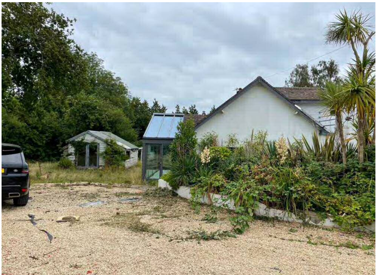
VIEW OF SIDE ELEVATION FROM THE SITE ENTRANCE-PREVIOUS PORCH EXTENSION VISIBLE
