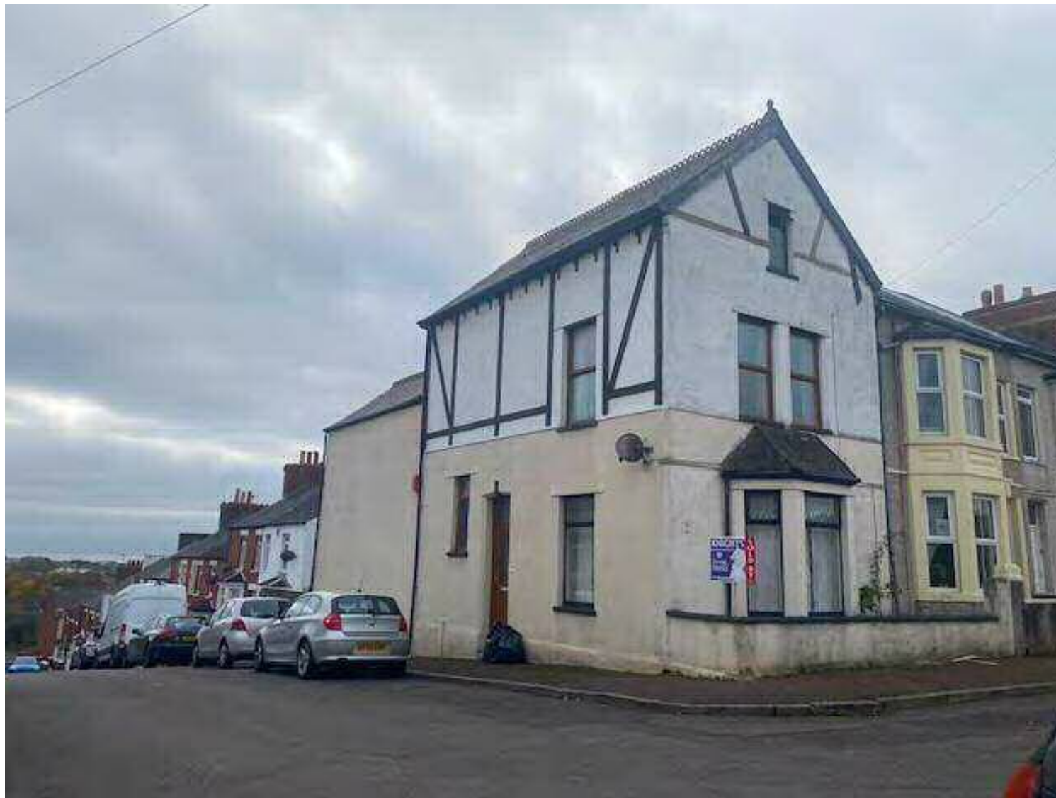
Site Photograph 1 – No 1 Rectory Road, Barry
