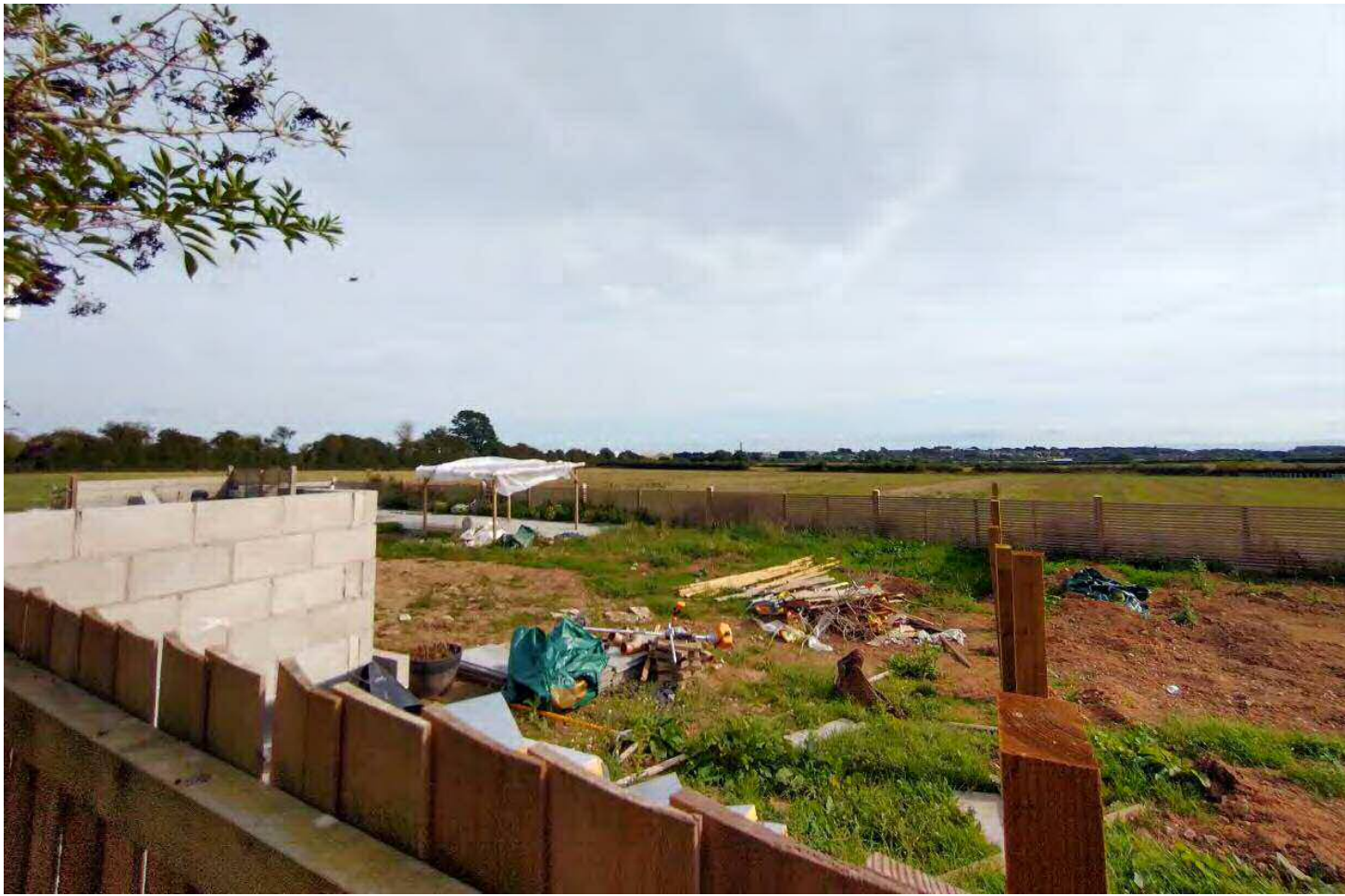
Site photograph 4 – view across site from neighbouring property
