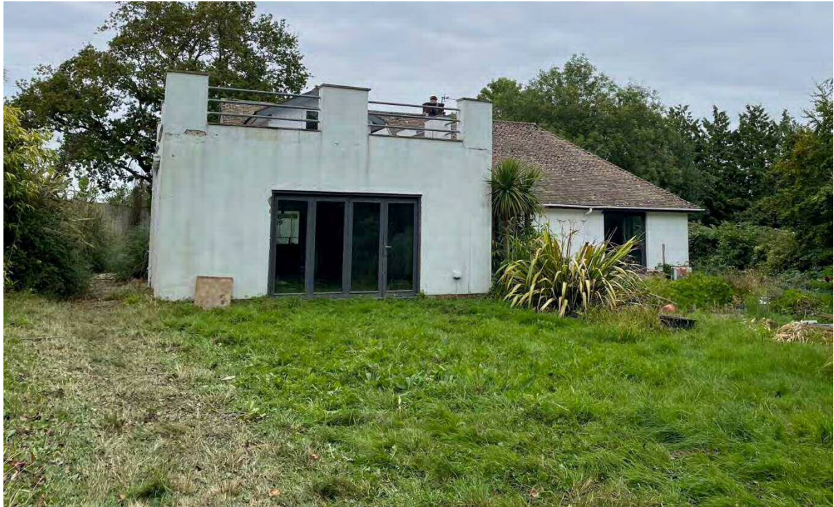
VIEW OF PPROPERTY TOWARDS THE REAR ELEVATION- PREVIOUS EXTENSION VISIBLE
