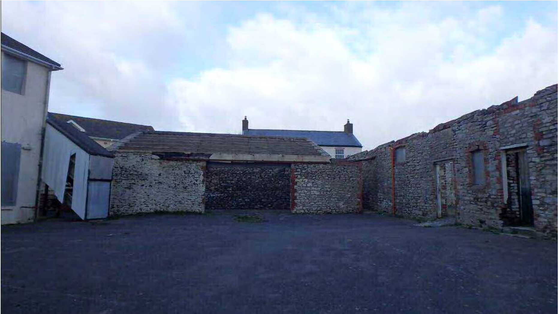
Site photograph 8 – site interior (dilapidated outbuildings)
