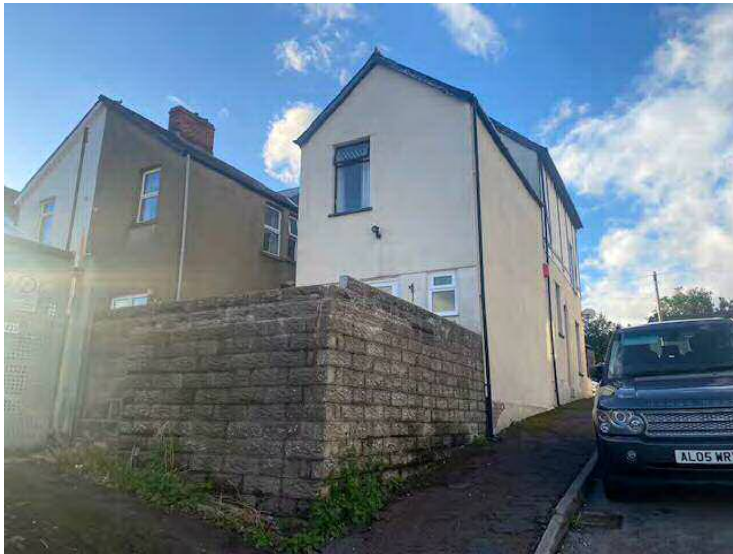
Site Photograph 2 – Rear Elevation
