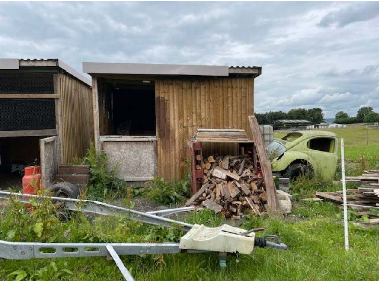
UNAUTHORISED SITING OF TRAILERS AND FIREWOOD
