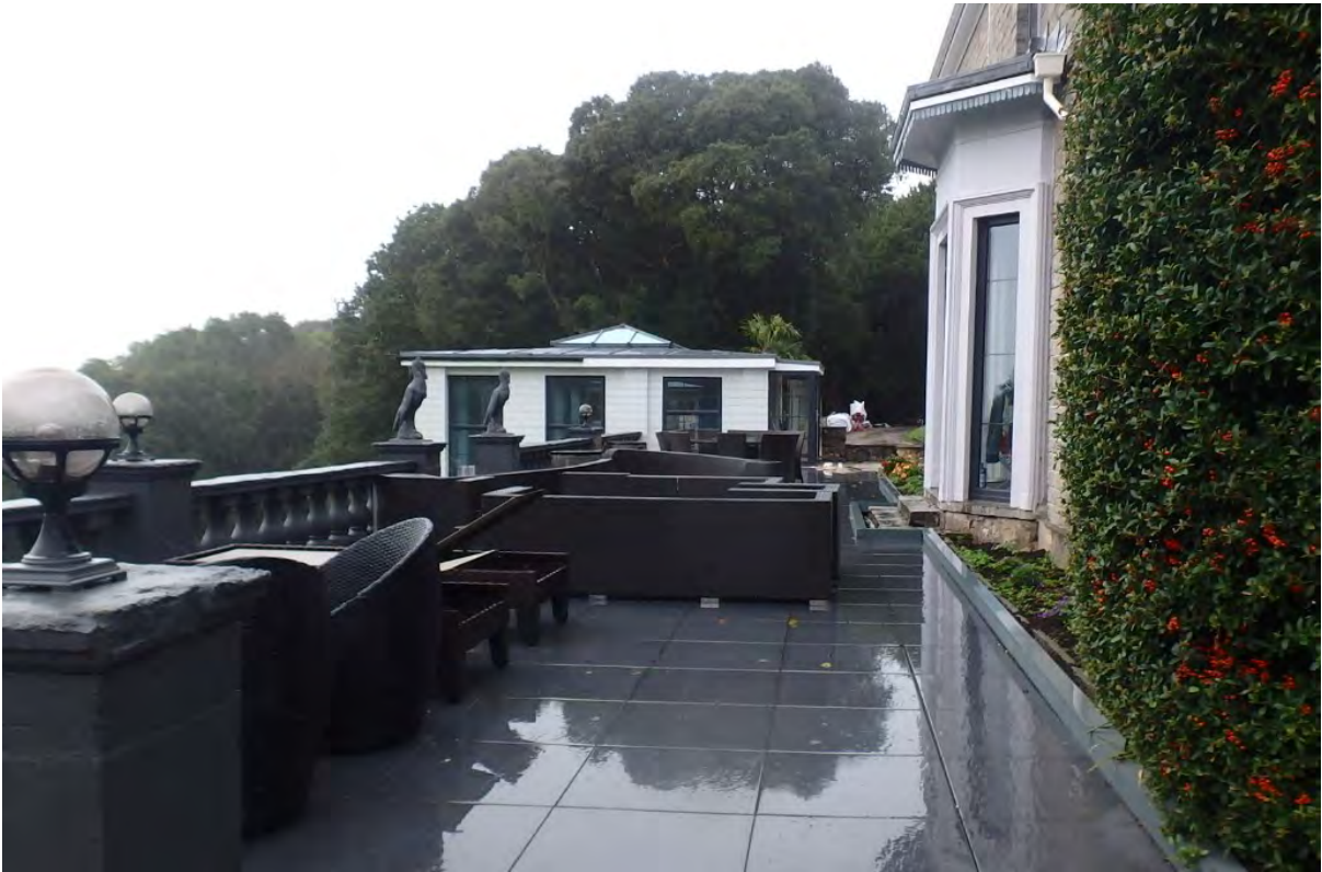
Pool house from the east
