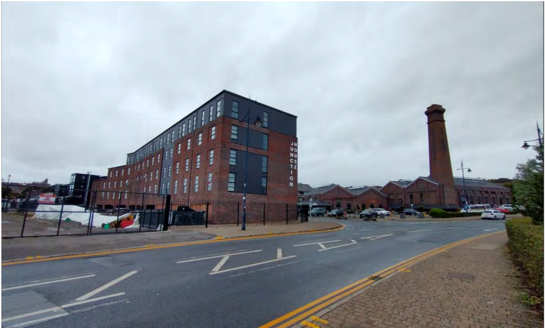
Site photograph 1 – view of Junction House from Hood Road
