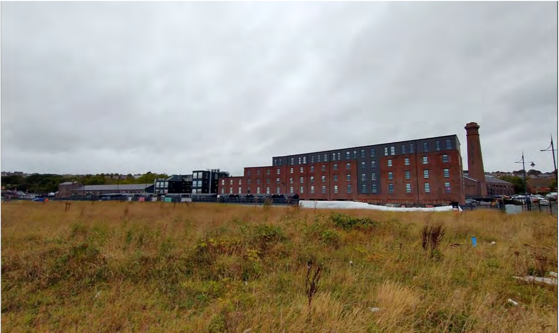
Site photograph 2 – view toward rear of Goodsheds site from Hood Road
