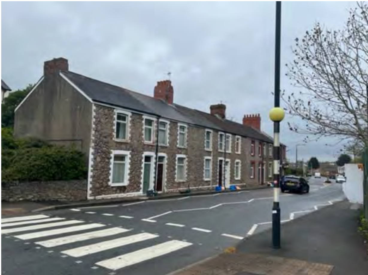
Site Photograph 3 – Neighbouring Terraced Dwellings (Coldbrook Road East)
