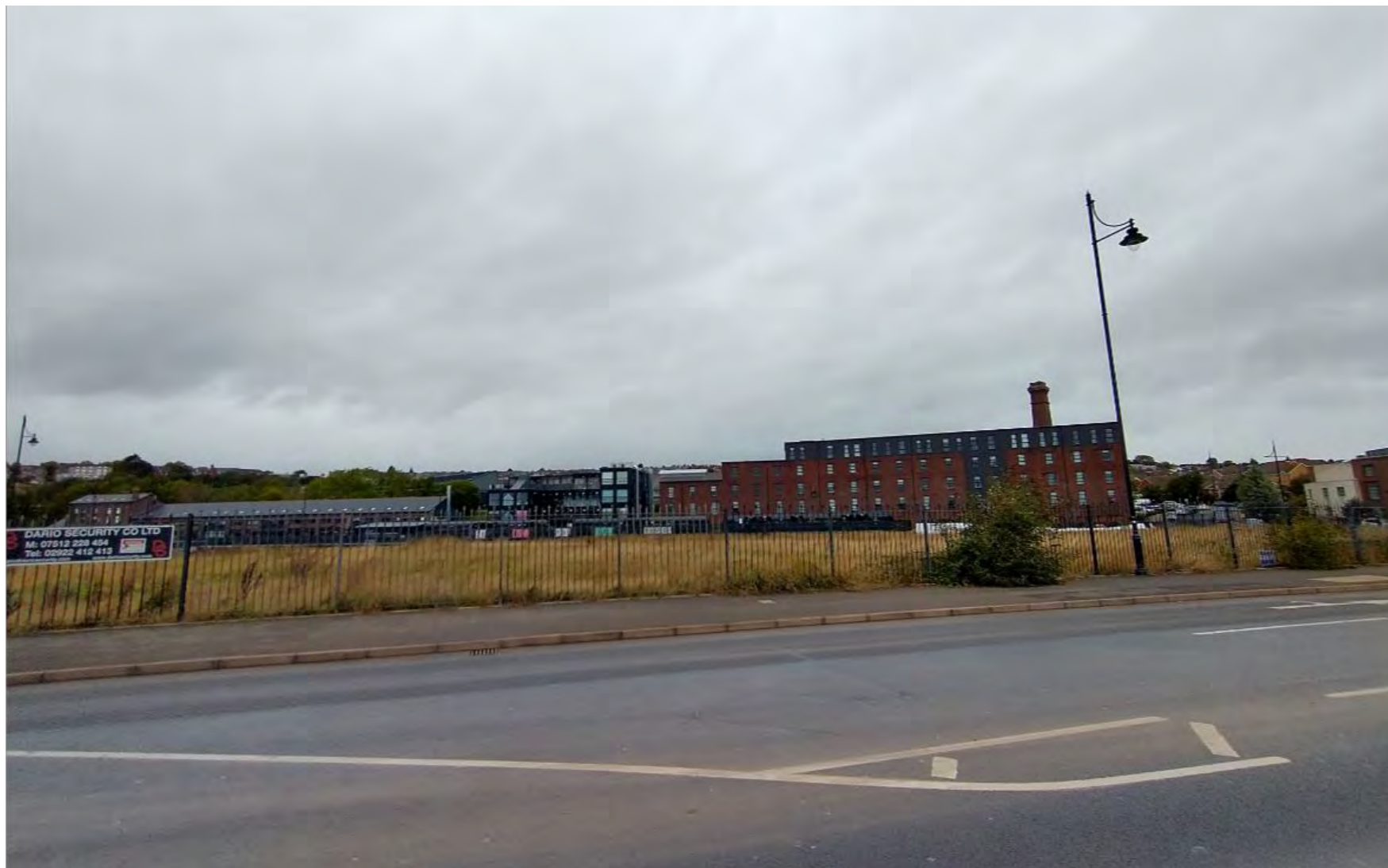
Site photograph 3 – view toward rear of Goodsheds site from Ffordd y Mileniwm
