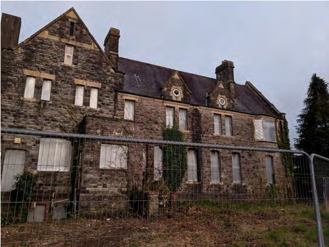
North-west facing elevation of the 1896 part of the building.
