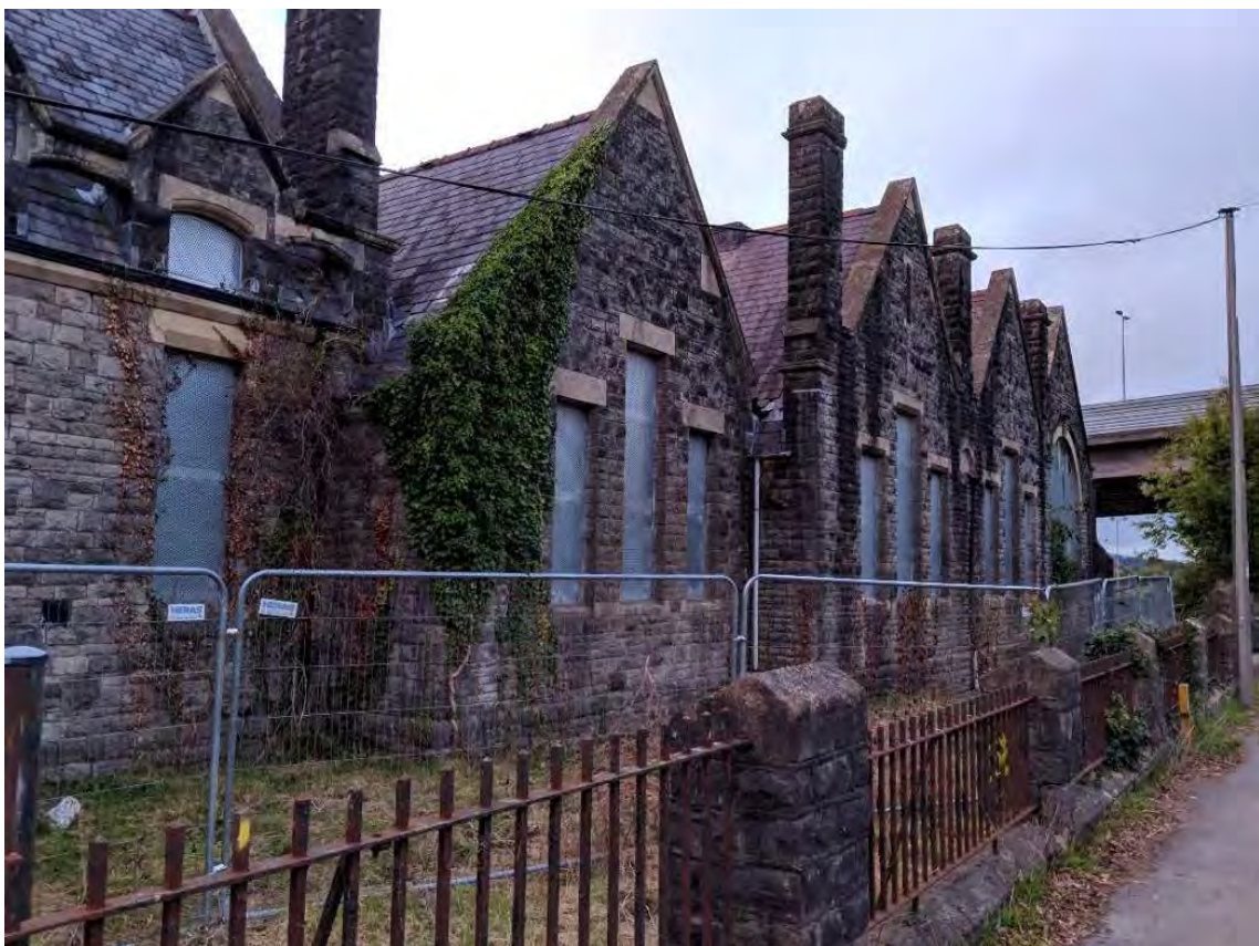
South-east facing elevations of the north-east end of the school building
