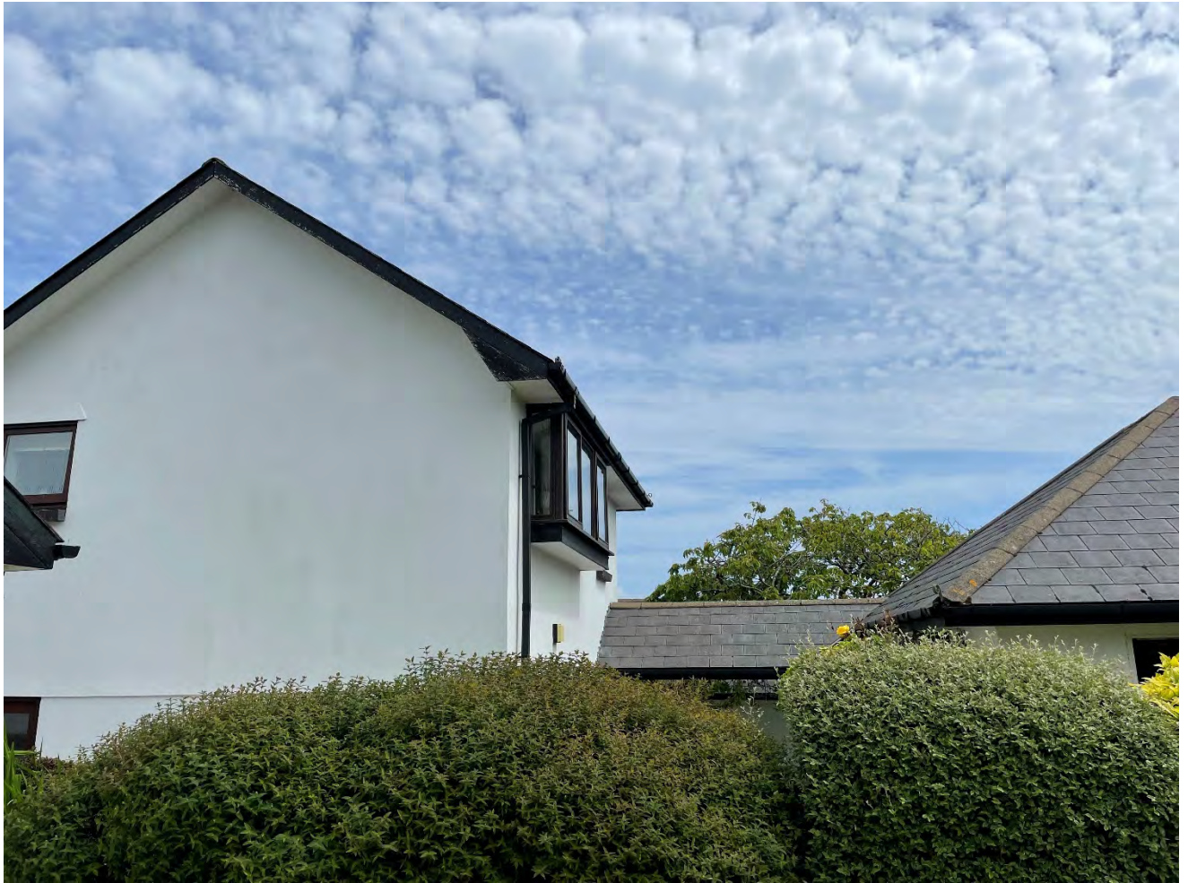
Site Picture 9: Outlook of the applicants' property from front/side garden at neighbouring property – 1 White House.
