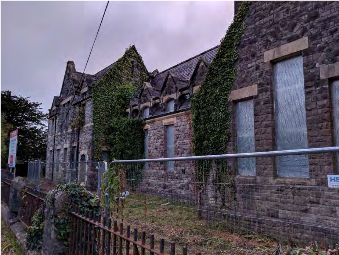
South-east facing elevations of the south-west end of the school building
