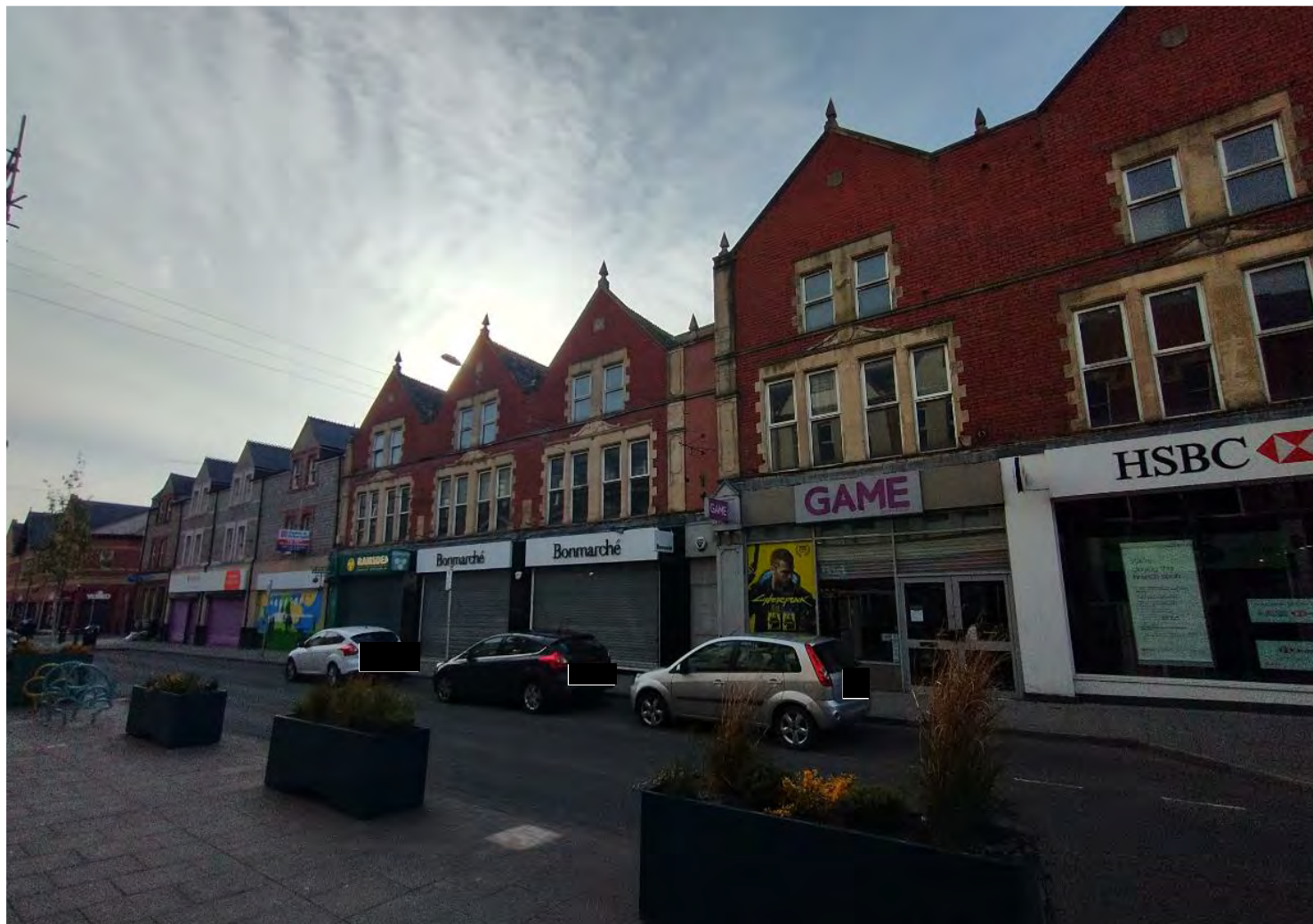
Site photograph 6 – front of building (Holton Road)
