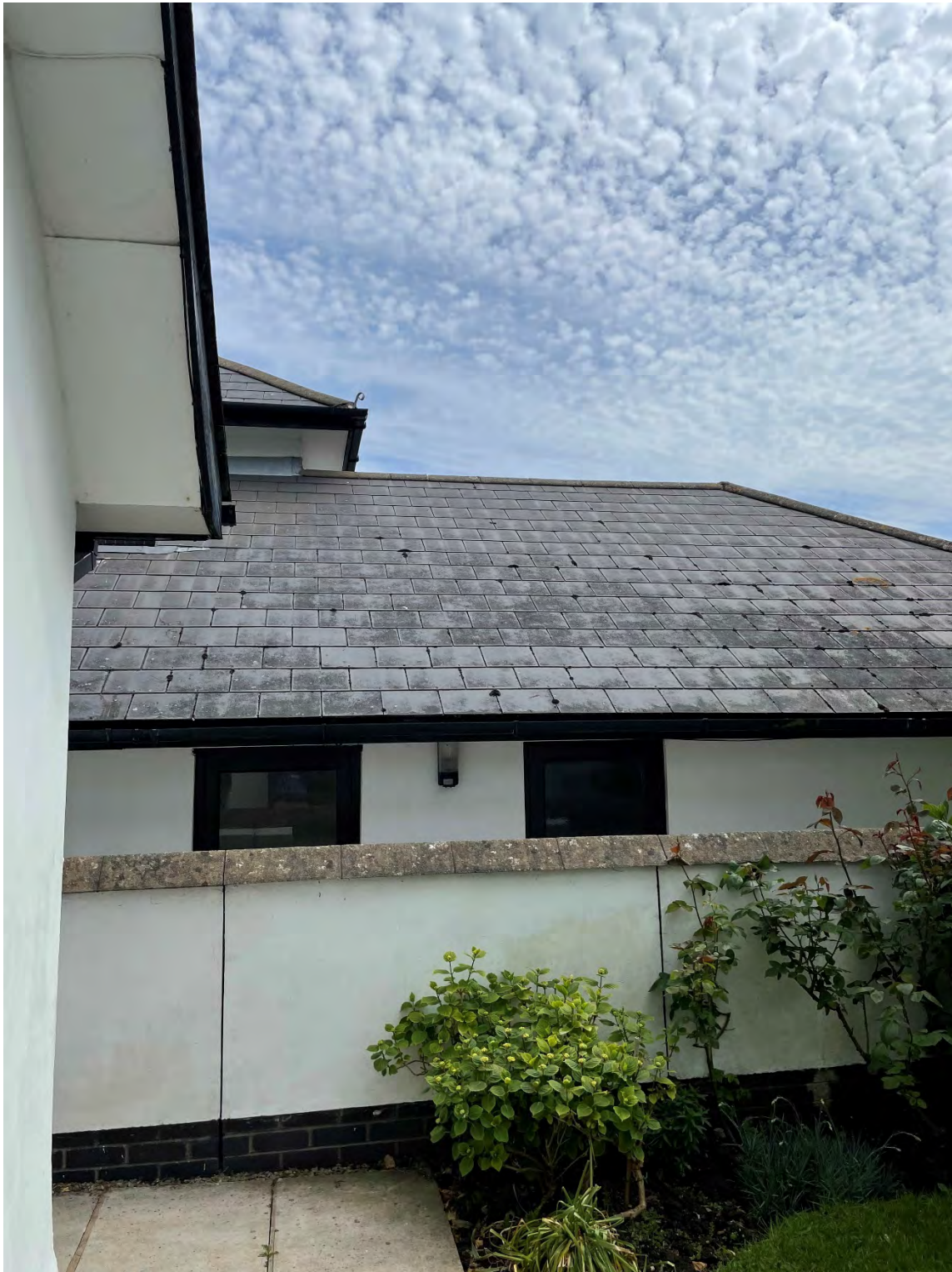
Site Picture 6: Picture from applicants' property eastwards facing neighbouring property – 5 White House.
