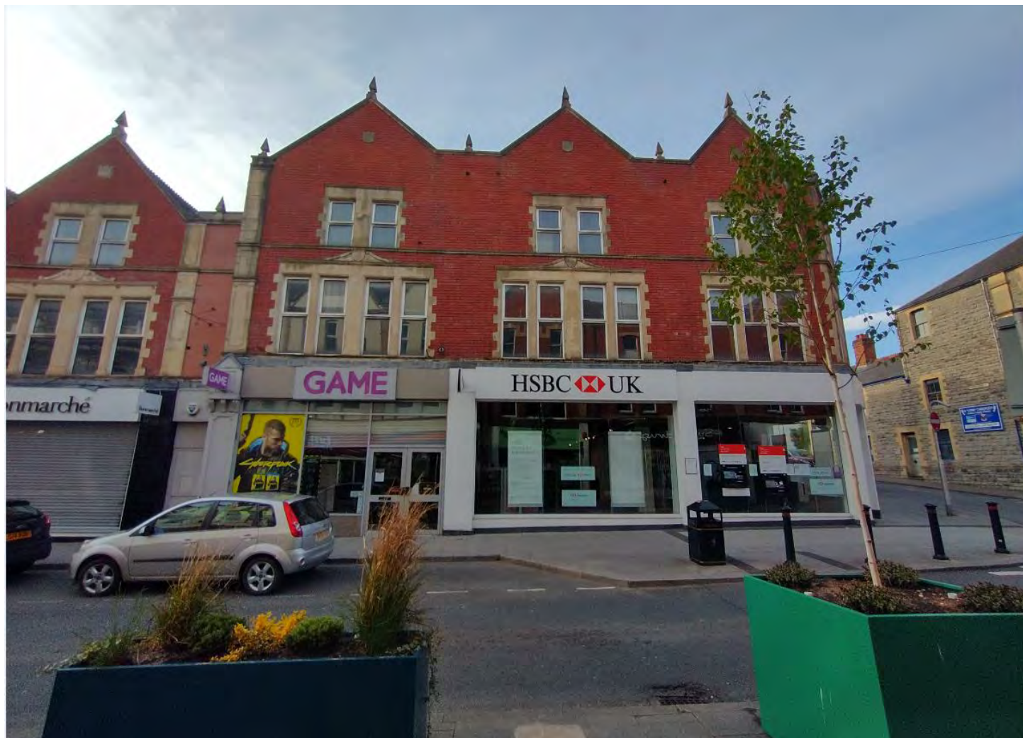
Site photograph 5 – front of building (Holton Road)
