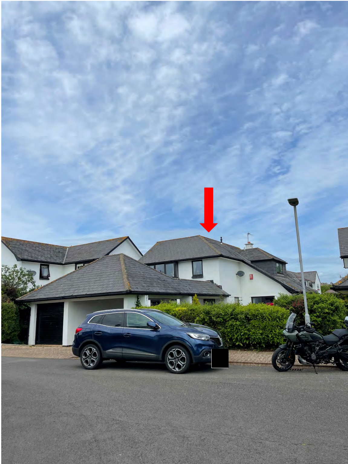
Site Picture 4: View of the application property (arrowed in red) from the street scene.
