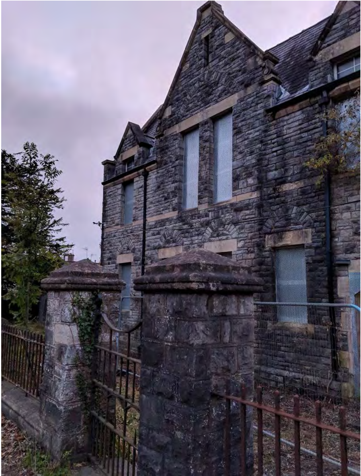
Facing gable on the south-east elevation.
