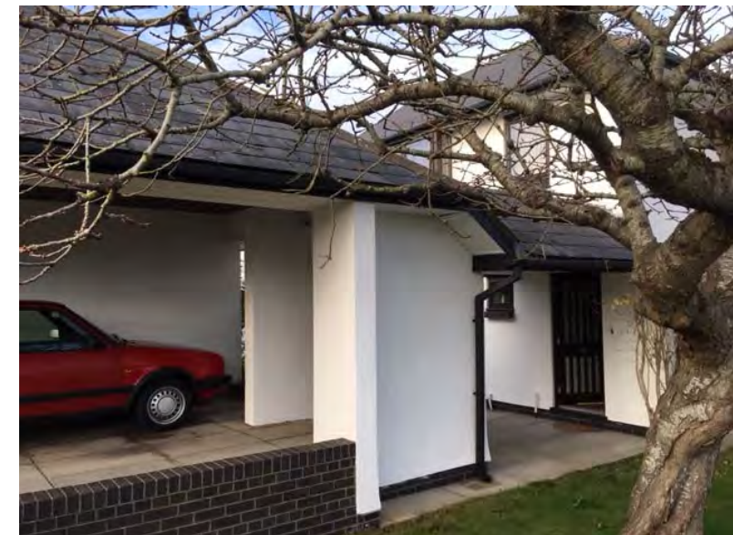
Deep soffit Feature
