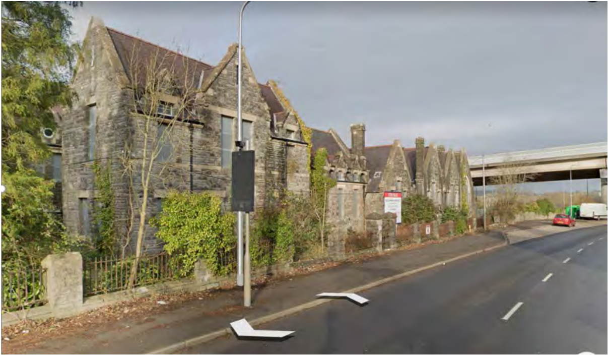
View from Aberthin Road looking North towards flyover
