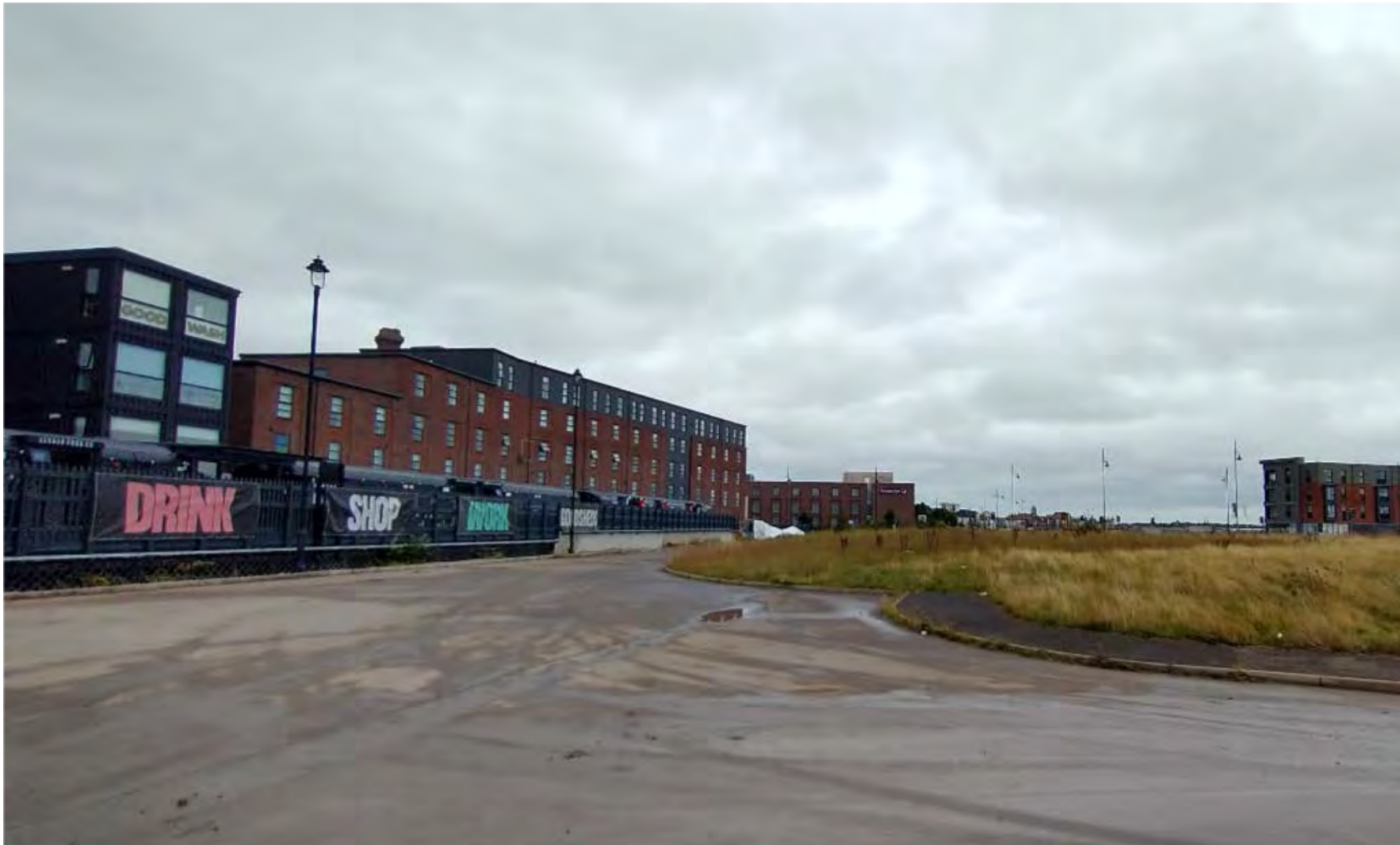
Site photograph 5 – view toward rear of Junction House from land at the south
