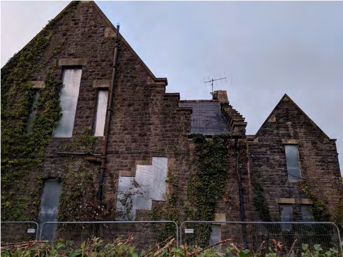
South-west facing elevation of the school building
