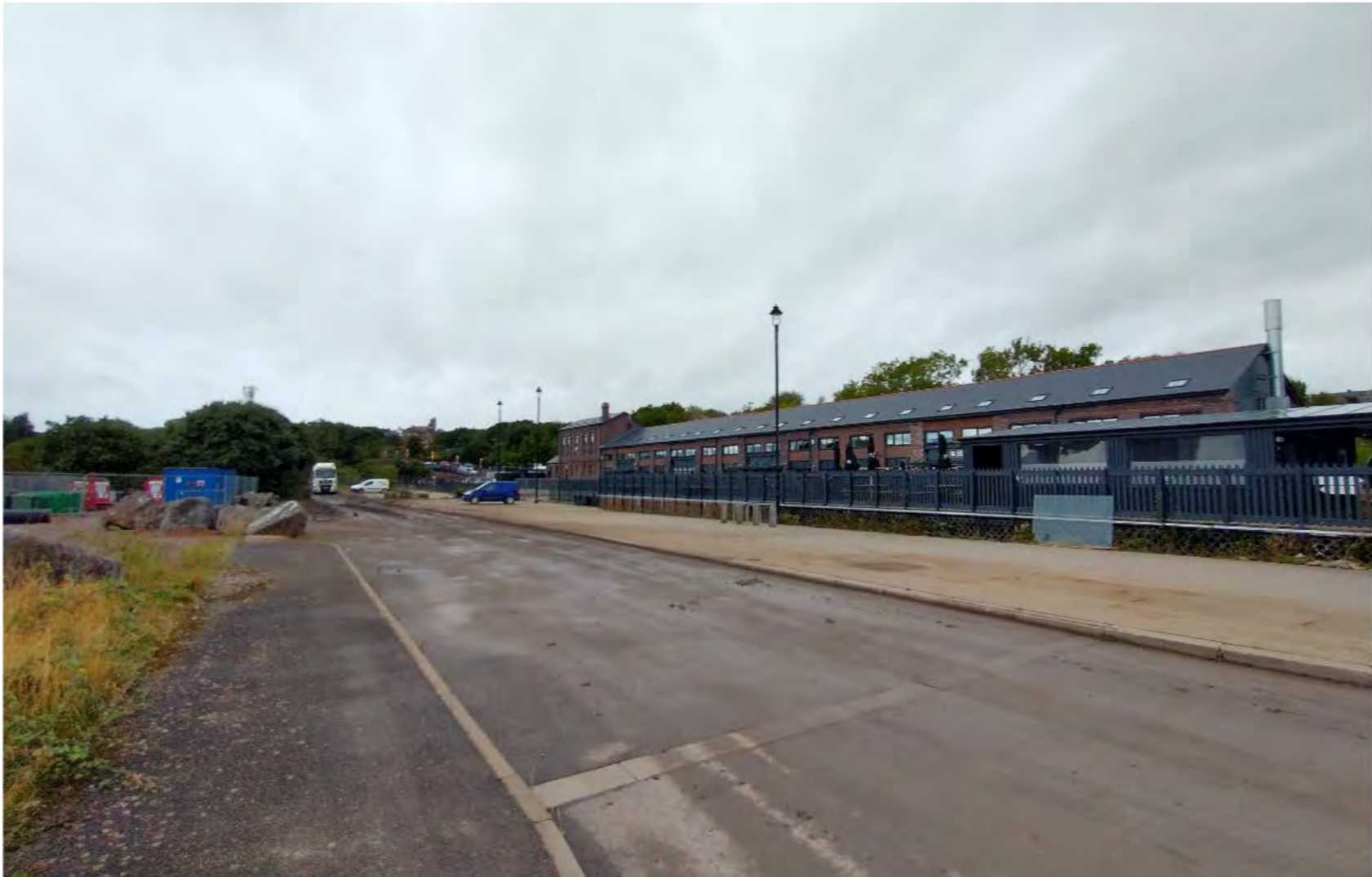
Site photograph 4 – view toward rear of Goodshed building from land to the south
