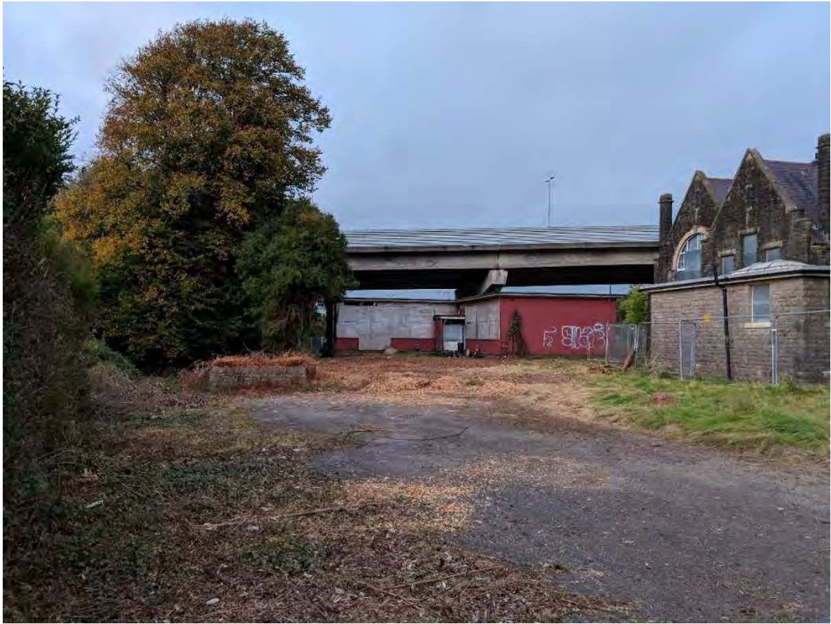
Rear of site - two remaining 1950s buildings and the stone wall remnant of the older outbuilding
