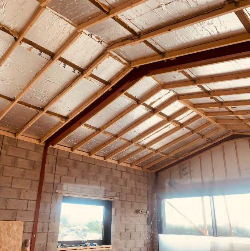
Interior Photographs of Barn F (November 2021):
