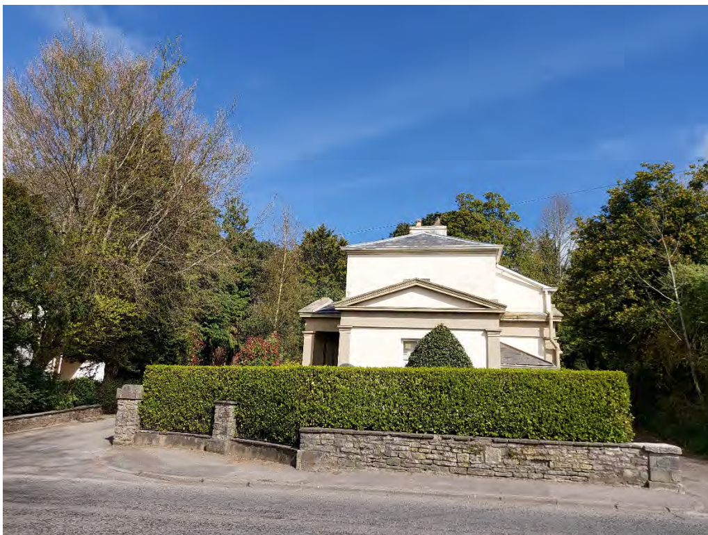
VIEW OF ADJOINING DWELLING FROM A48
