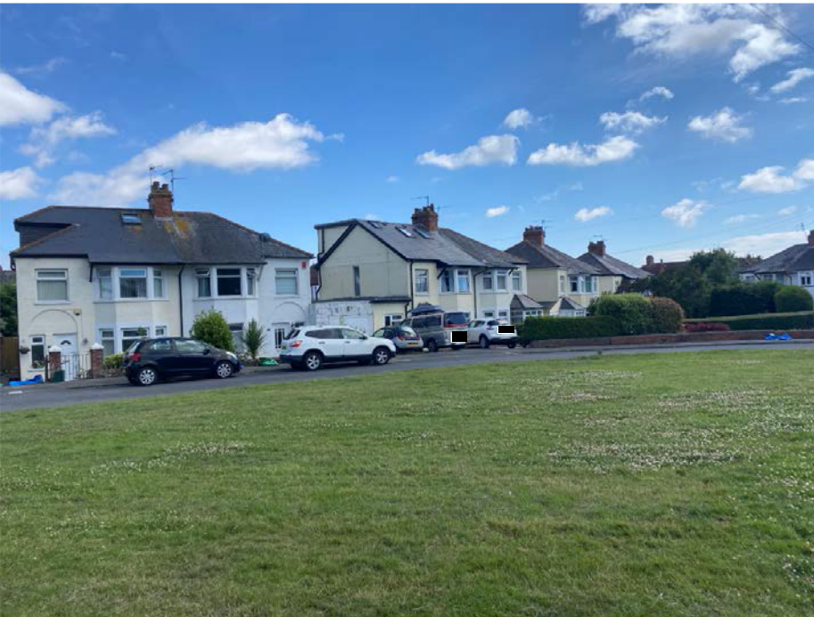
Figure 2: Image of dwelling within Mountjoy Crescent with a hip to gable alteration and rear dormer
