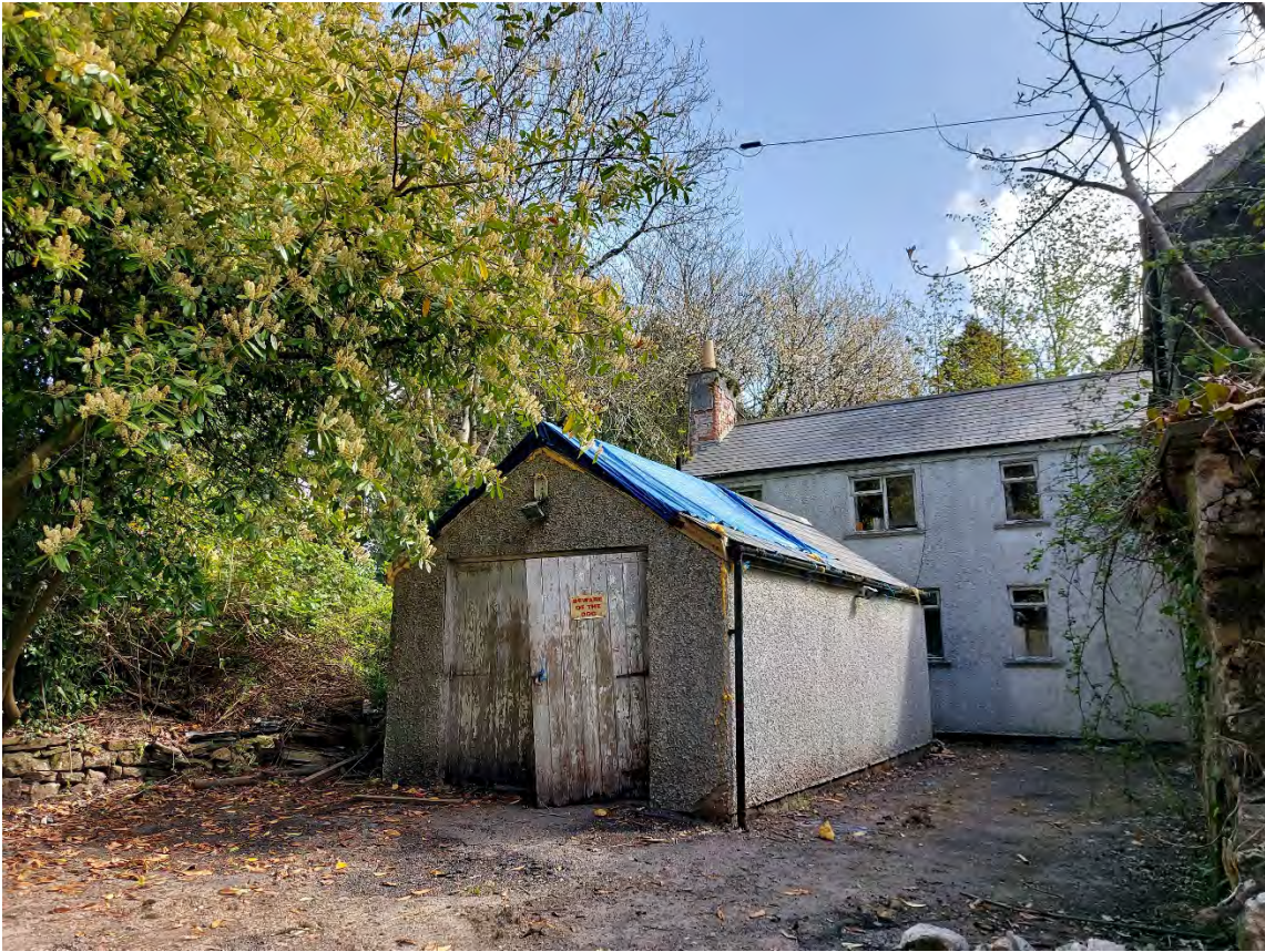
VIEW OF EXISTING GARAGE
