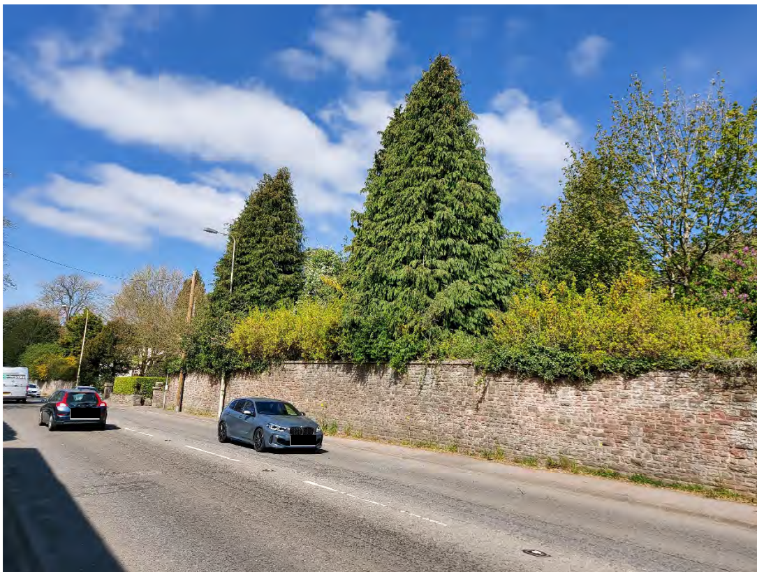
VIEW OF WALL – LOOKING WEST TOWARDS ENTRANCE
