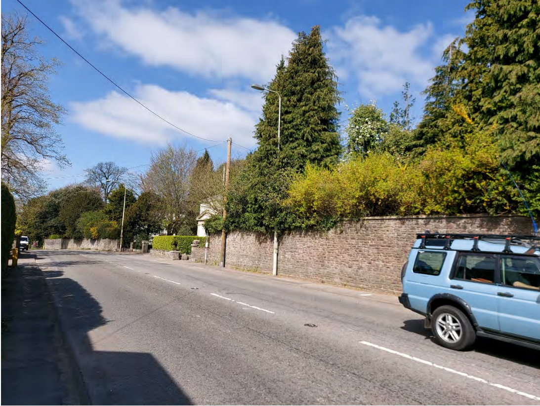
VIEW OF WALL – LOOKING WEST TOWARDS ENTRANCE
