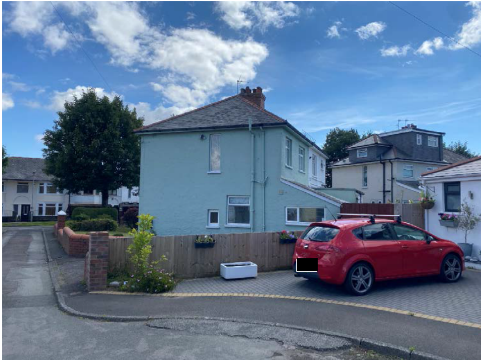
Figure 8: side elevation of the applicants dwelling from within Mountjoy Close, the image also includes the driveway of No7
