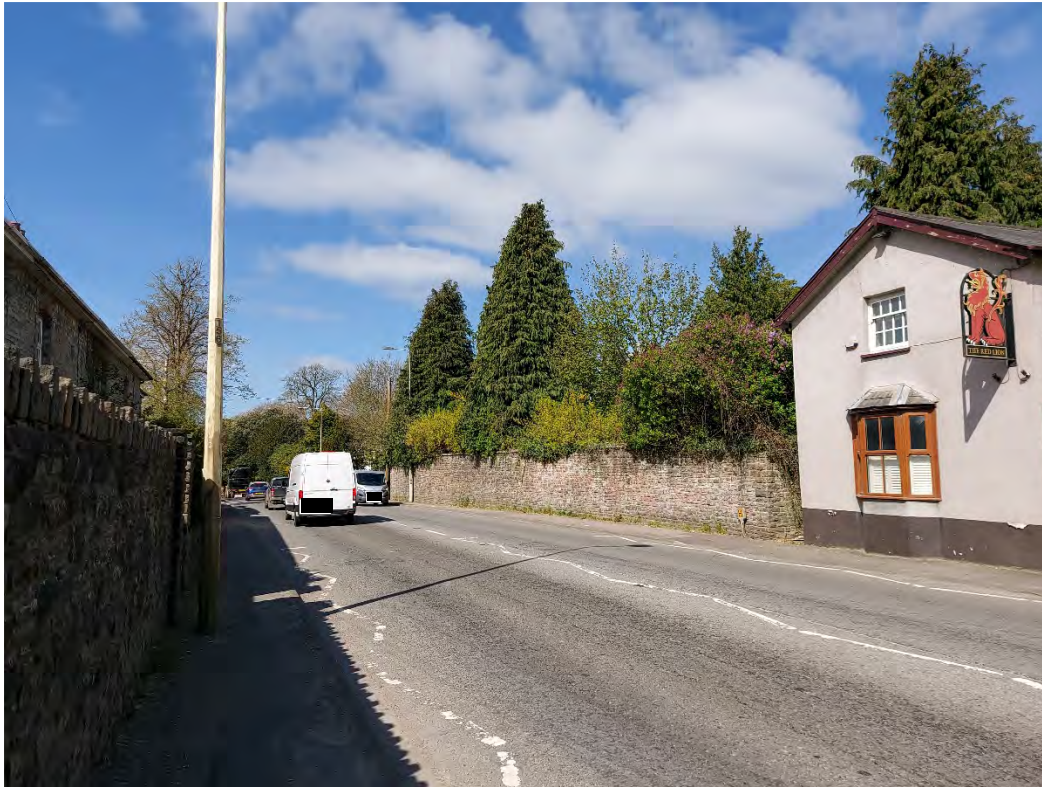
VIEW OF WALL – LOOKING WEST TOWARDS ENTRANCE
