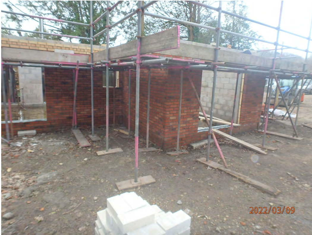
Building as partly constructed
