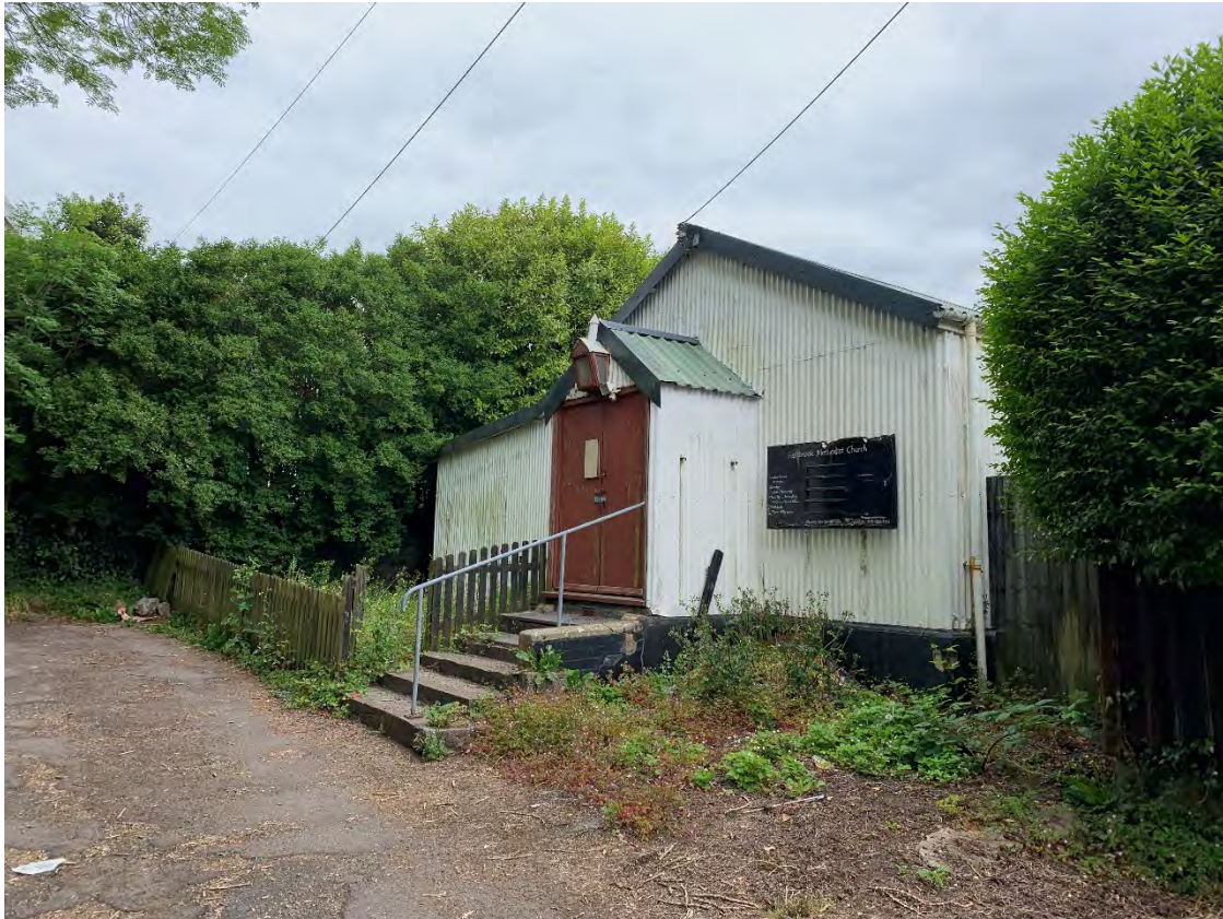
View of front elevation of Chapel
