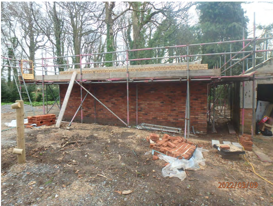
Building as partly constructed
