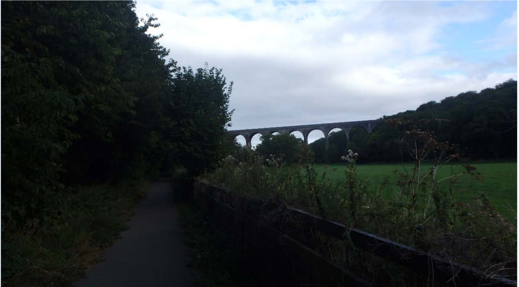
Site photograph 6 – view from Porthkerry Park toward viaduct/ site
