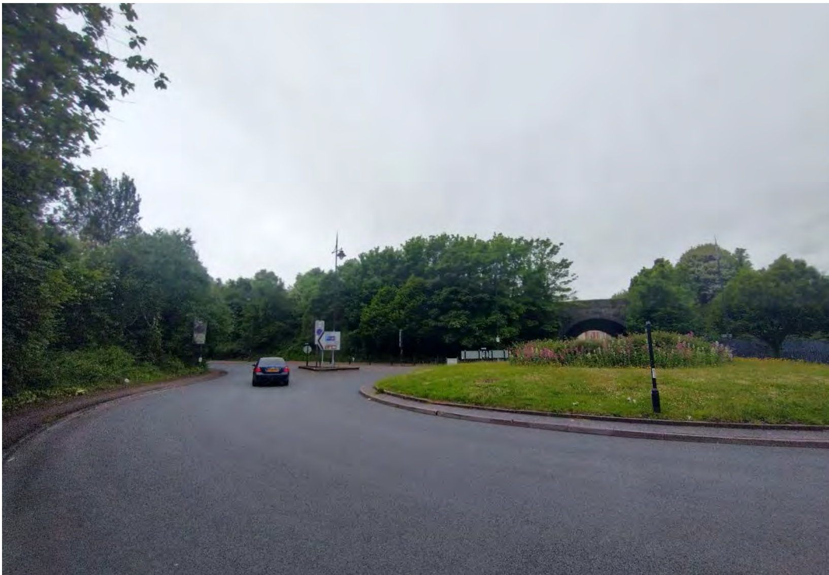
Site photograph – from Ffordd y Mileniwm/ Cardiff Road/ Gladstone Road roundabout
