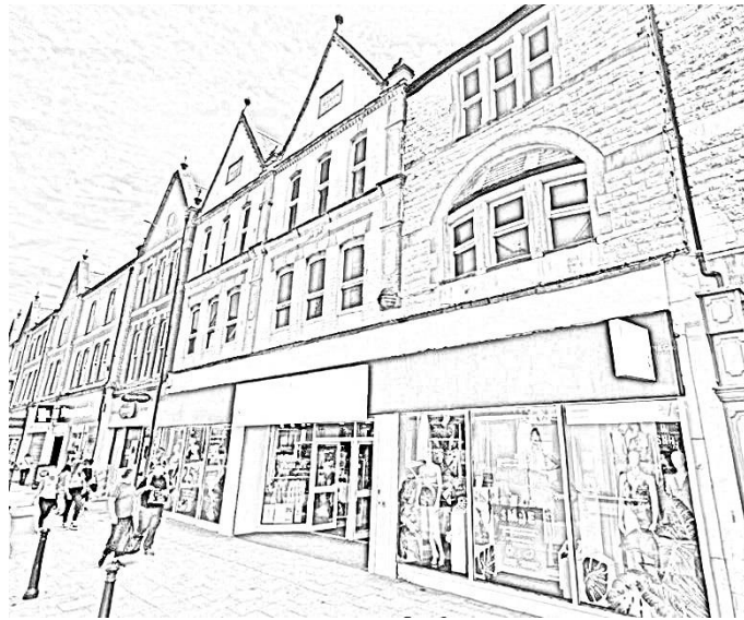
Figure 4: Example of Inappropriate Shop frontage for a Traditional Setting
