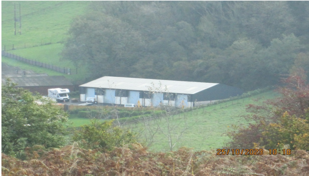
View of building from Stalling Down
