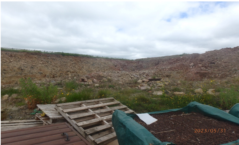
View of excavated area from the south-east
