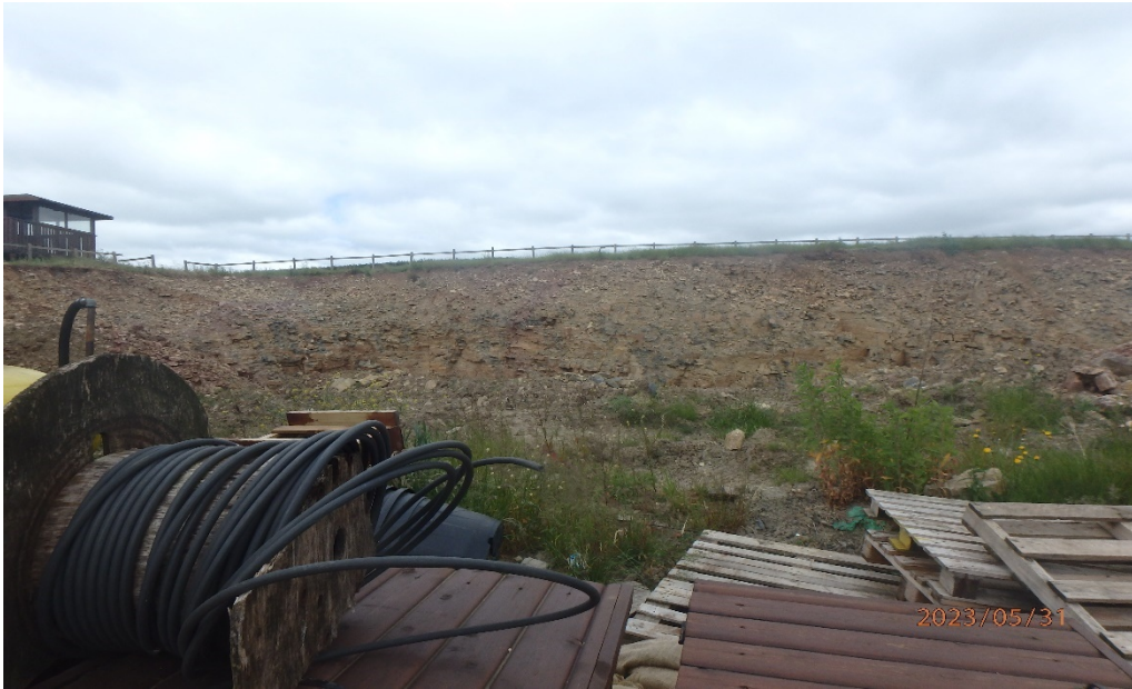
View of excavated area from the south
