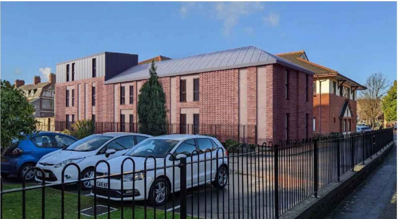
Third design iteration – 2 / 3 storey extension to south and west of the original building
