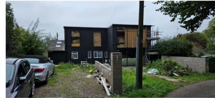
Photos of Front Elevation, as built.
