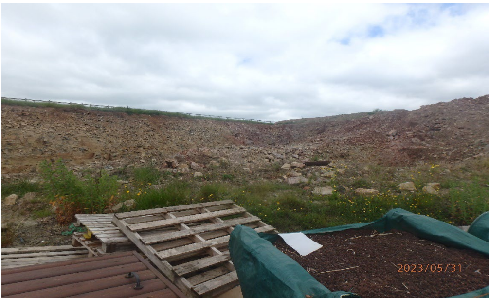
View of excavated area from the south-east
