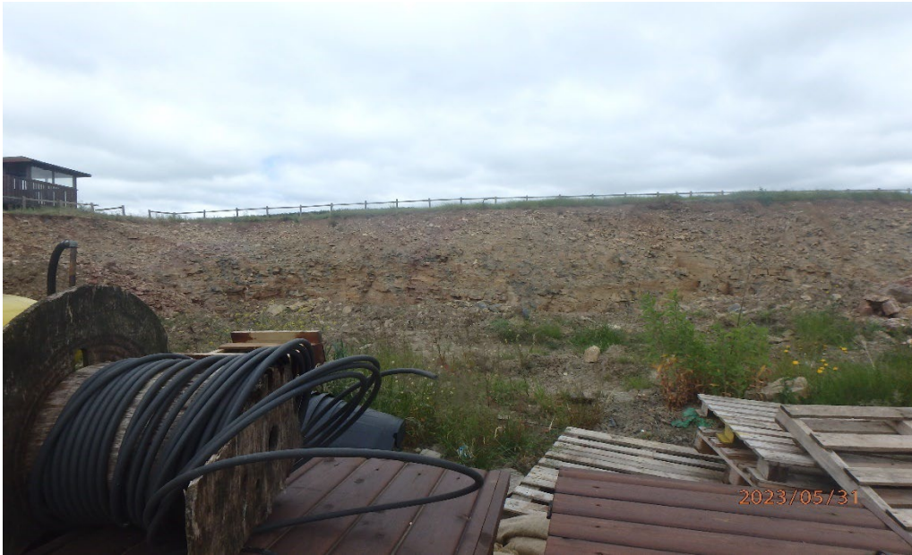
View of excavated area from the south
