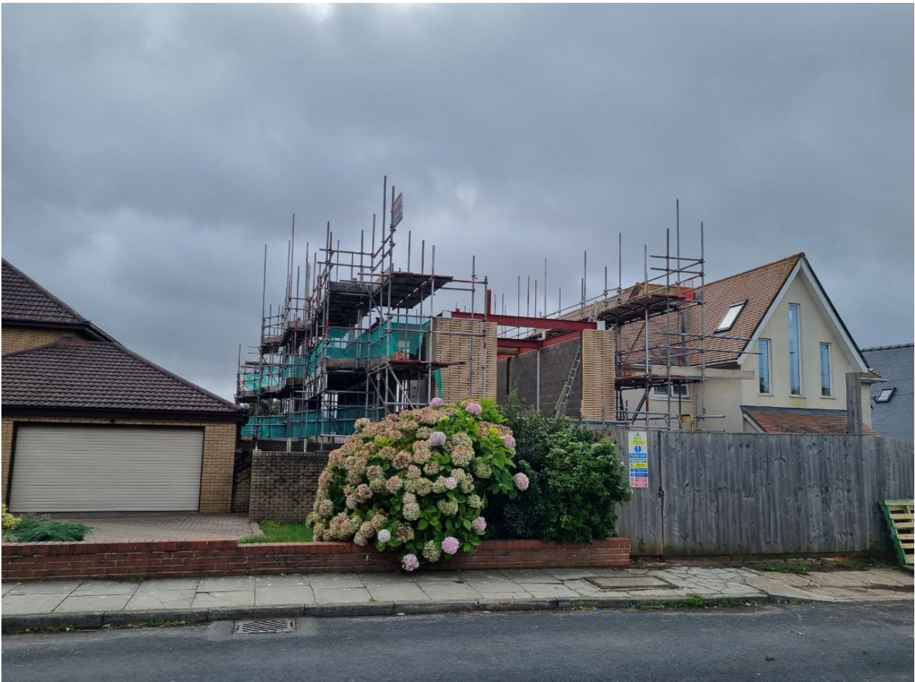
Part-built dwelling with scaffolding (September 2024)
